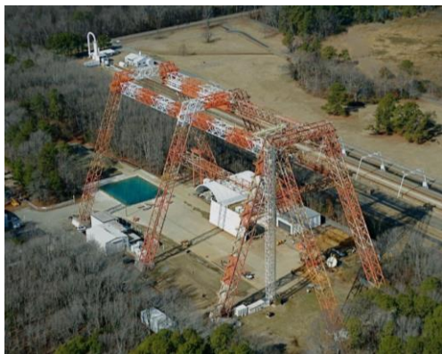
Landing and Impact Research Facility
