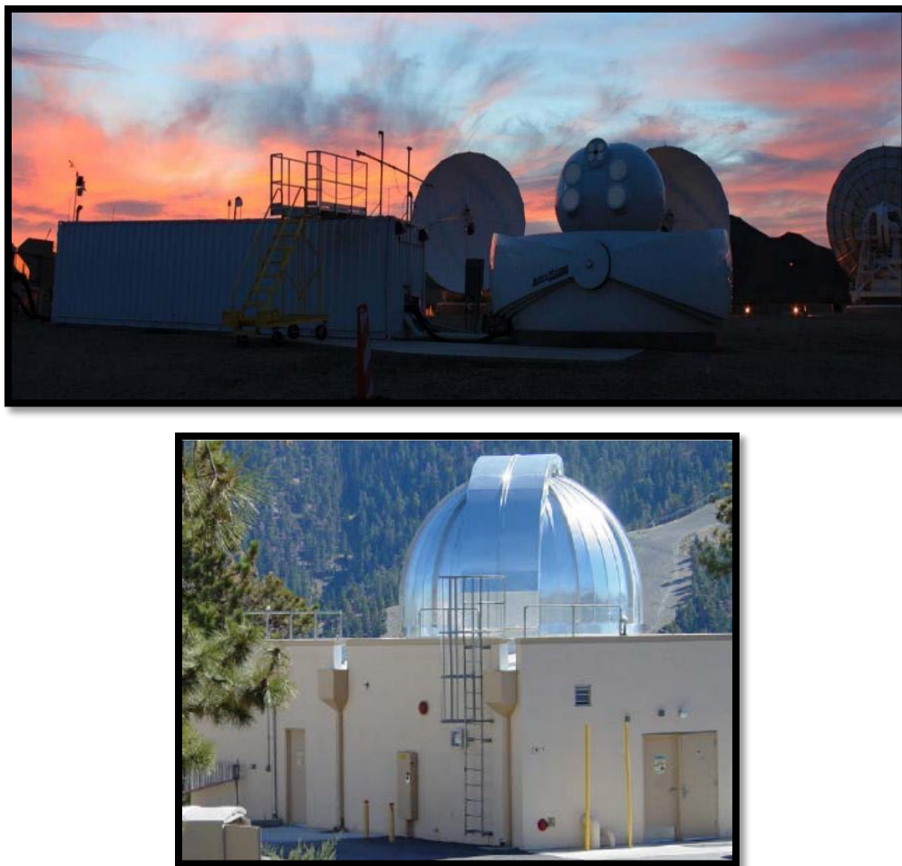
Figure 1. Top: Image of the LLGT at White Sands used to receive the 622Mbps downlink from the Lunar Laser Communication Demonstration (LLCD). Bottom: JPL's Table Mountain Facility used in many laser communication demonstrations such as LLCD and that will be used to receive the Laser Communication Relay Demonstration (LCRD) downlink.
