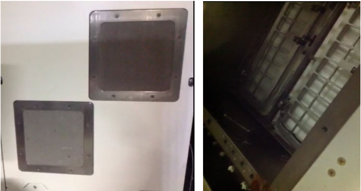
Figure 21. Good Grill Design (Left); these Grills are Highly Visible and Easy to Access and Clean. Poor Grill Design (Right); This Grill is Hard to Access for Cleaning and Requires Tools.
