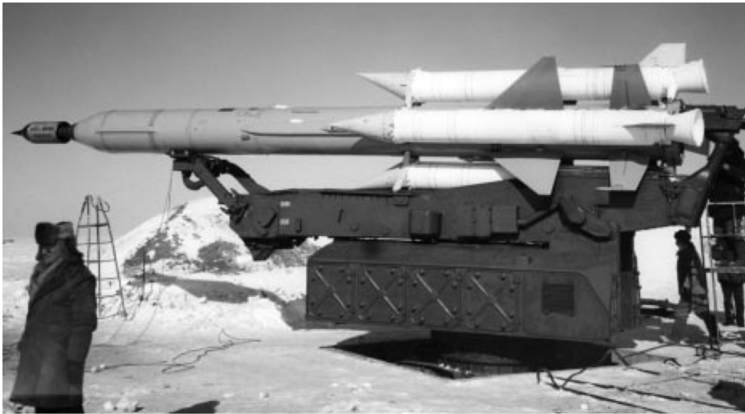
Figure 8. The SA-5 booster and HFL launch configuration.
