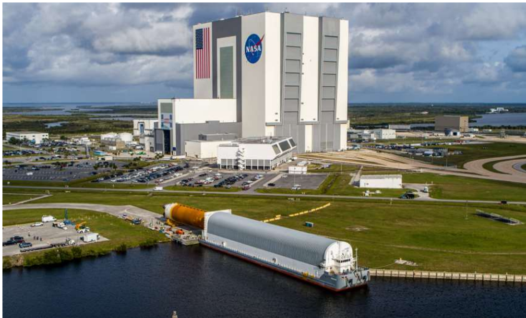
Figure 1. Space Launch System (SLS) core stage arriving to KSC [10]
