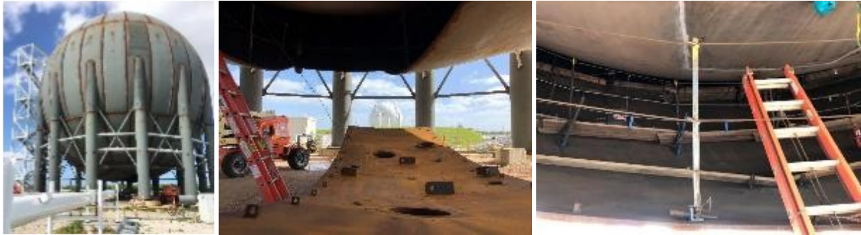
Figure 7. New LH 2 tank under construction: overall view with VJ transfer line (left); final plate section for external shell (middle); and view of annular space (right).
