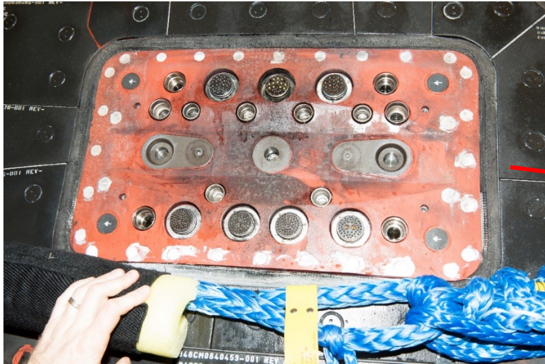
Charring of RTV on Umbilical Panel
