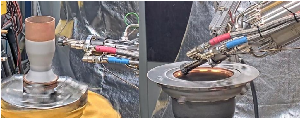
Figure 8. Cold spray of bimetallic chamber structural jacket (left) and cold spray repair of bimetallic chamber (right).
