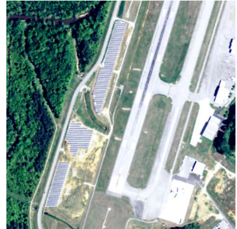
Solar arrays outside of runway object free area at Chattanooga Airport (CHA)
