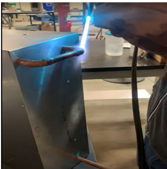
Figure 24 Brazing fittings to the piping system
