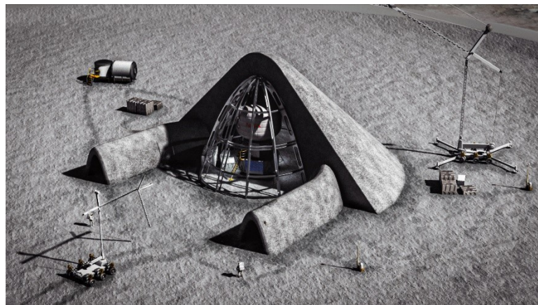
Figure 5. Artist's rendition of LSH Baseline Concept 1.1A: Metallic structure with regolith overburden to protect surface habitat – Cutaway view. Structure shown is notional and for illustration purposes.
