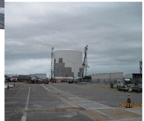
Tank Being Insulated
