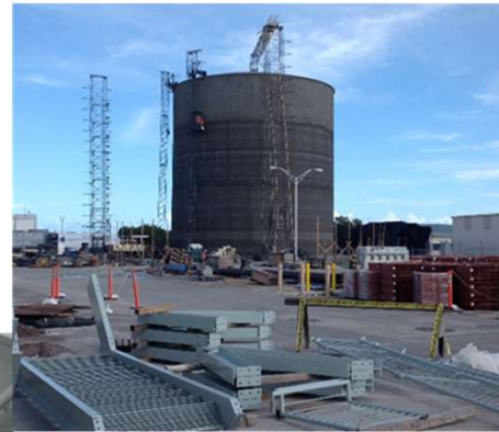
Tank Being Wrapped
