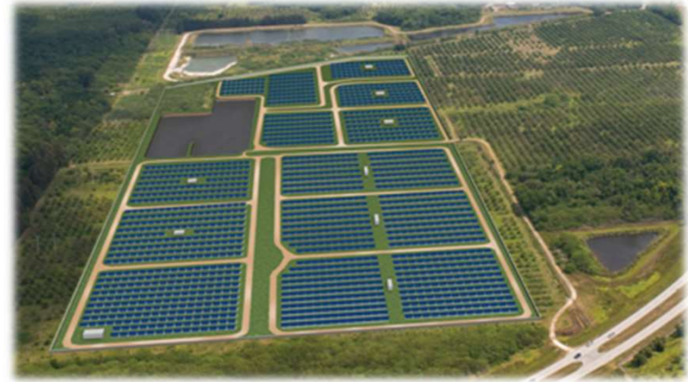
Space Coast Next Generation Solar Center
