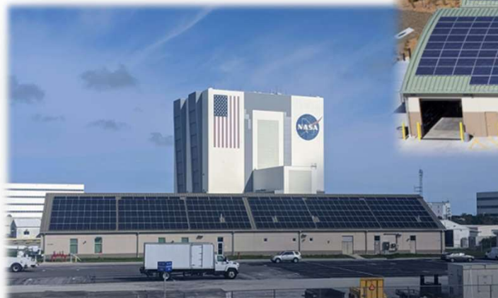
Electrical Maintenance Facility
