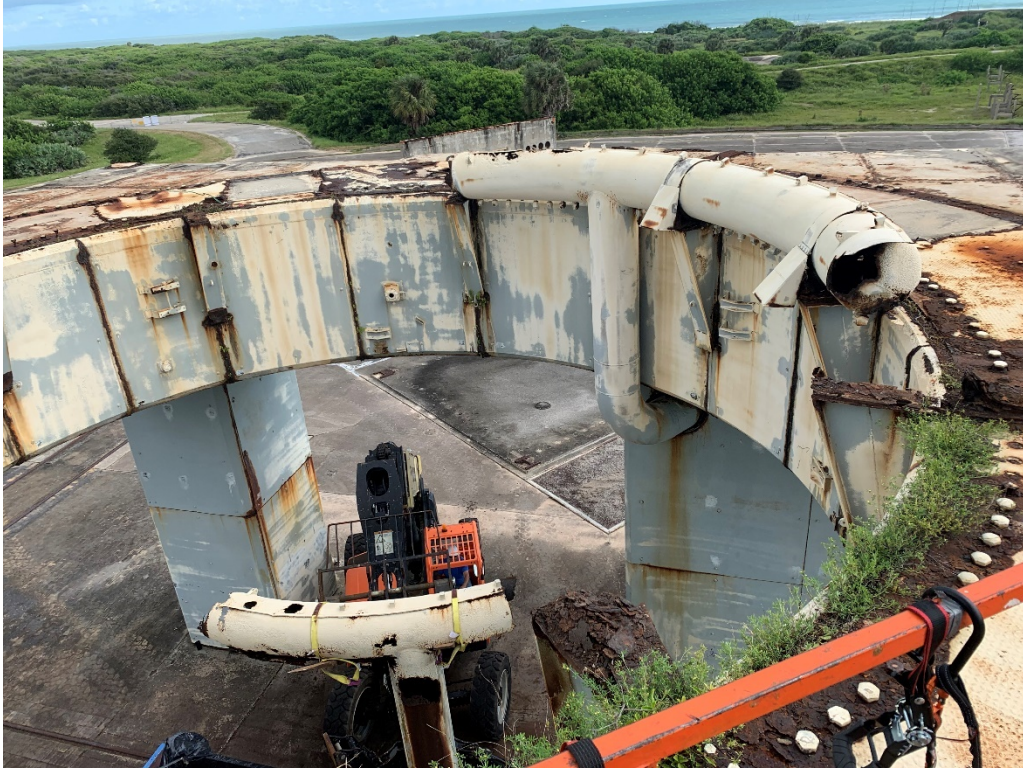
Figure 41: 9/16/2020 10:19:40 AM; lowering Torus Ring section and down pipe
