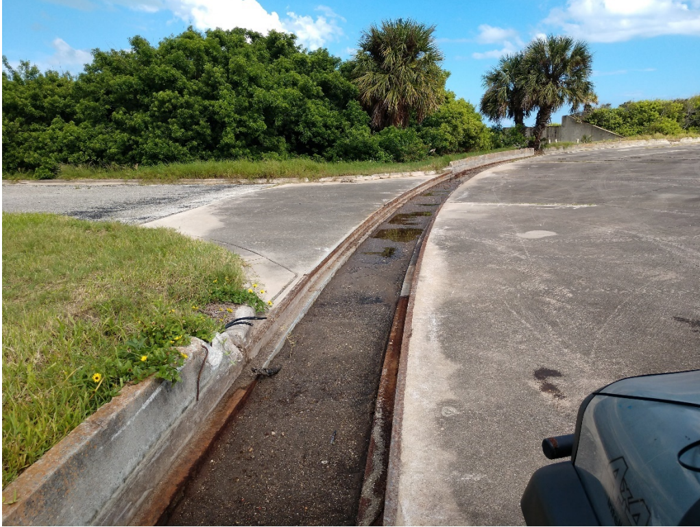
Figure 83: 9/29/2020 3:20:49 PM; facing NE, excavated trench on N side of launch pad
