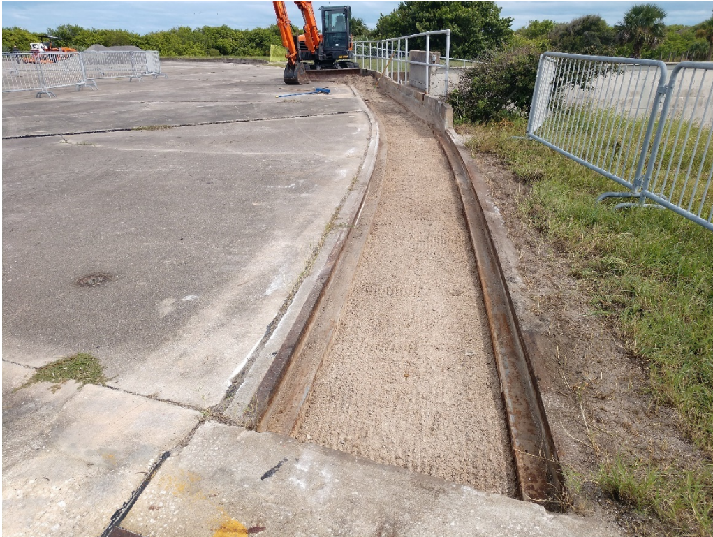
Figure 113: 10/1/2020 3:09:58 PM; facing E, excavated trench on S side of launch pad
