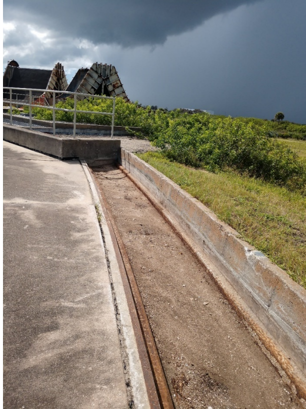
Figure 81: 9/29/2020 3:19:45 PM; facing W, excavated trench on NW side of launch pad
