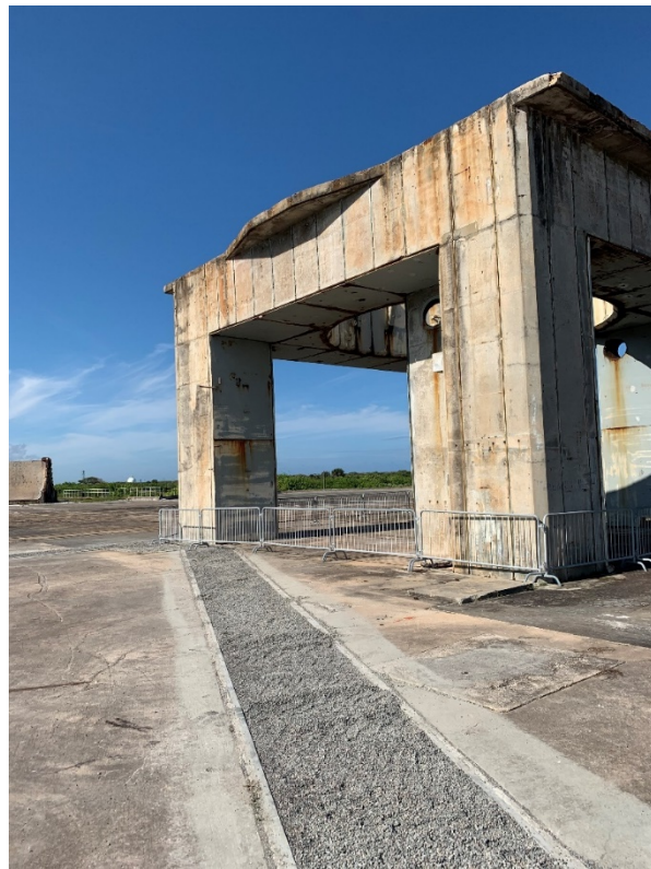
Figure 132: 10/8/2020 3:35:20 PM; facing N, launch pad and Pedestal following restoration activities
