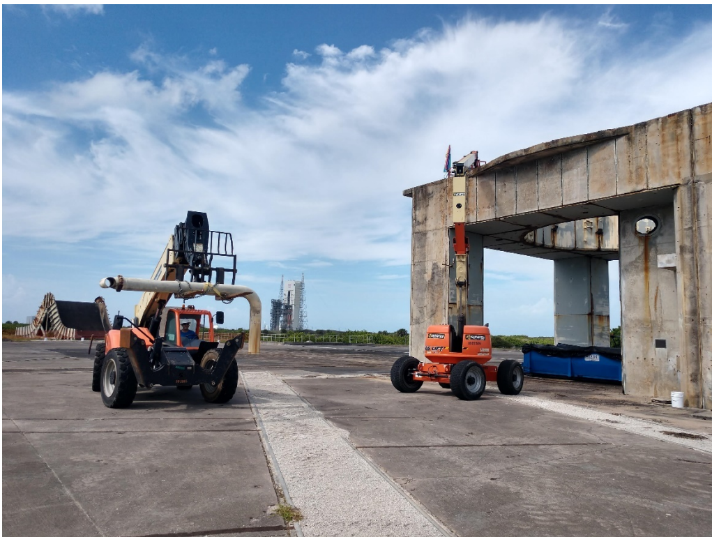
Figure 64: 9/24/2020 3:18:23 PM; removed feed pipe being transfer to roll-off box
