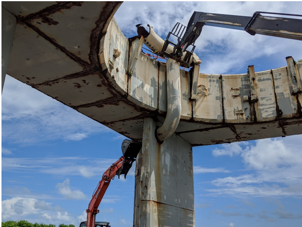
Figure 46: 9/16/2020 1:47:50 PM; removing Torus Ring section and down pipe
