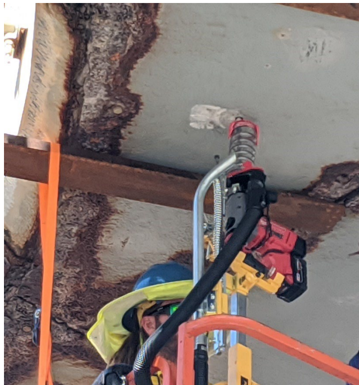
Figure 4: 9/9/2020 10:25:28 AM; drilling hole for anchor installation
