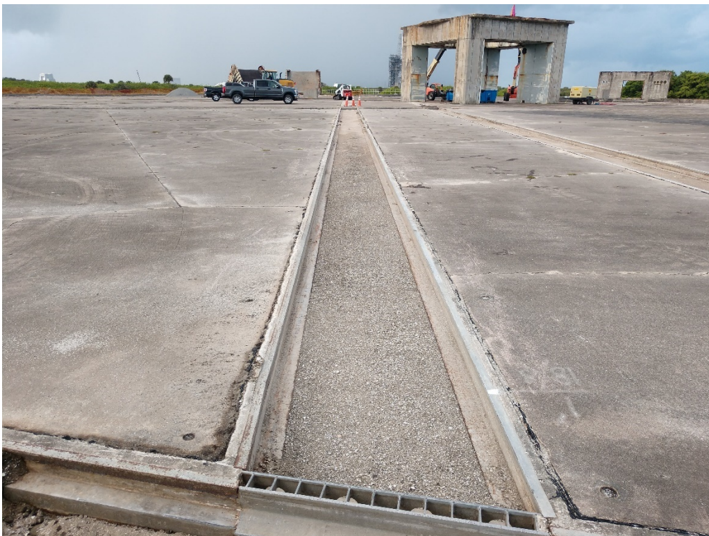
Figure 98: 9/29/2020 3:27:32 PM; facing NW, excavated trench on S side of launch pad
