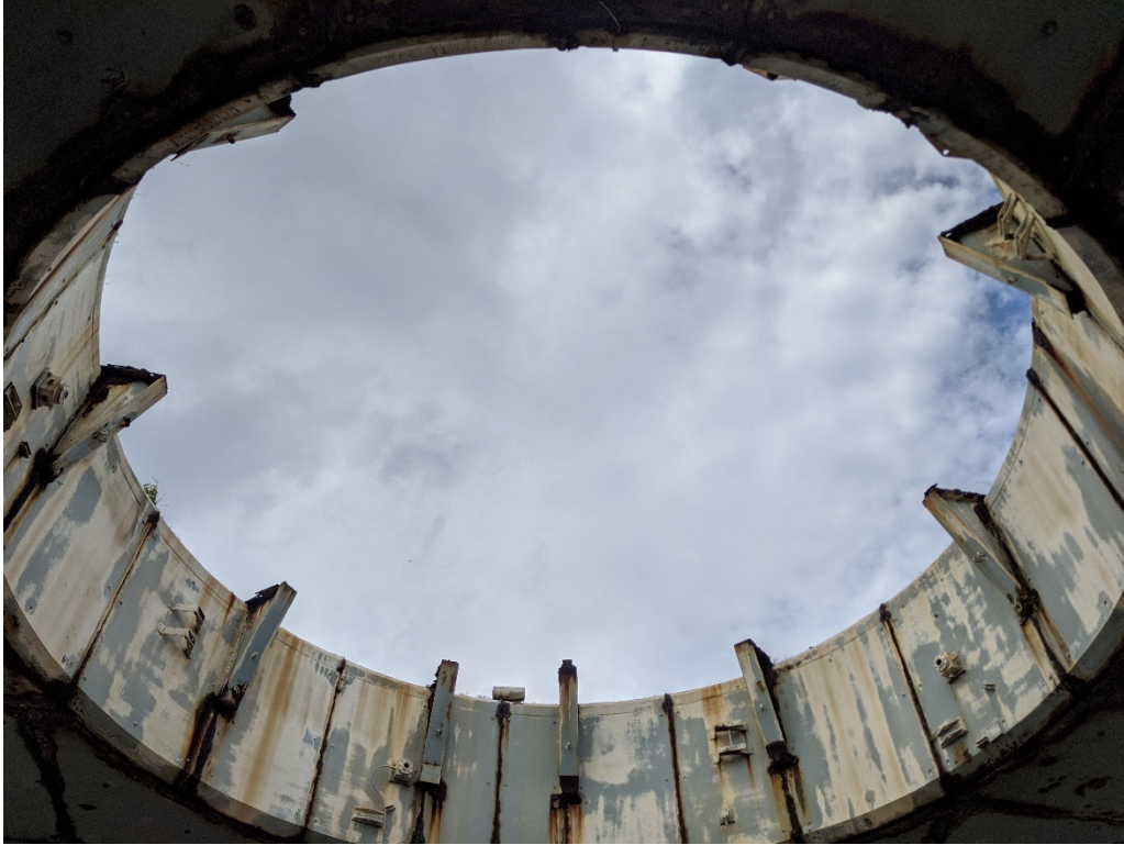
Figure 51: 9/16/2020 2:17:54 PM; looking from underneath Pedestal with Torus Ring removed
