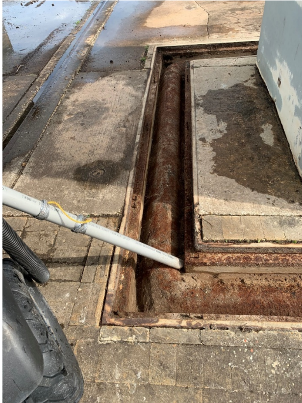
Figure 129: 10/5/2020 3:41:23 PM; vacuuming trenches
