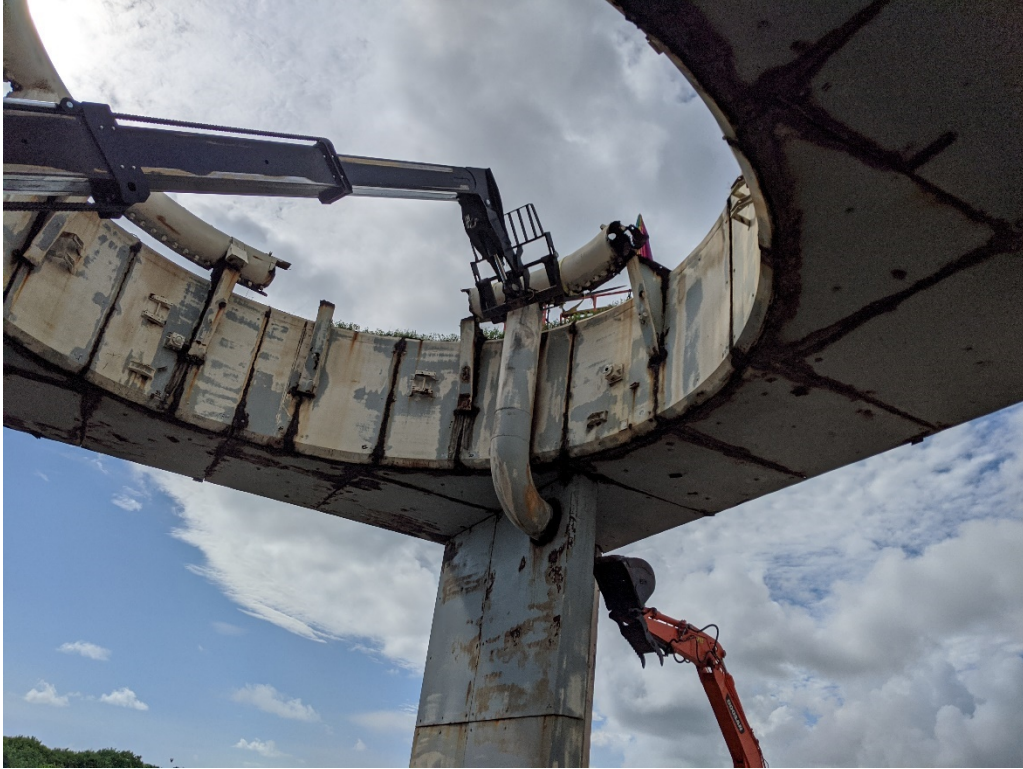
Figure 39: 9/16/2020 10:16:59 AM; removing Torus Ring section and down pipe
