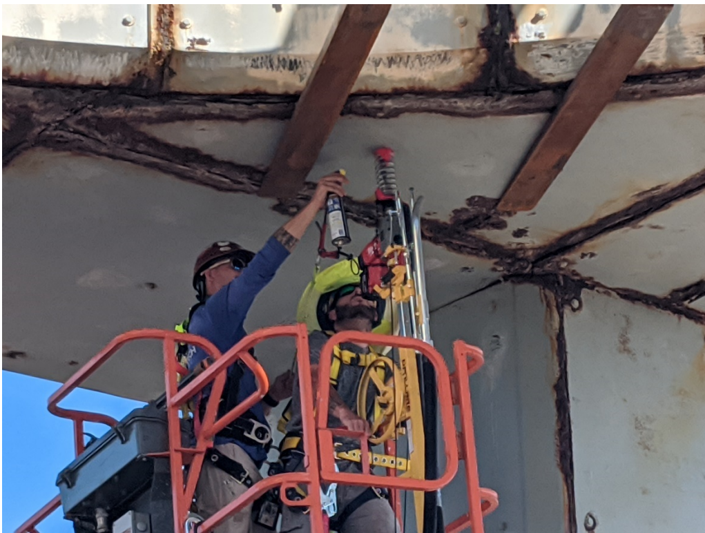
Figure 2: 9/9/2020 10:05:40 AM; drilling hole for anchor installation
