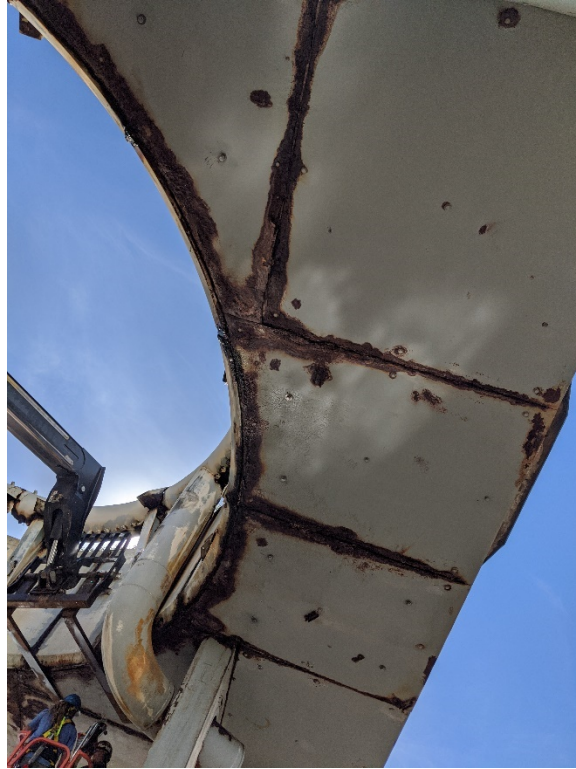
Figure 13: 9/11/2020 10:14:20 AM; looking at underside steel plates with newly installed anchors
