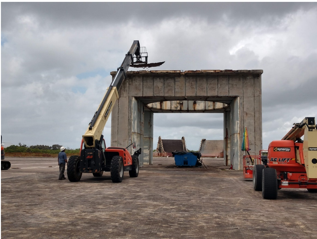
Figure 60: 9/24/2020 11:29:26 AM; removing top side steel plates
