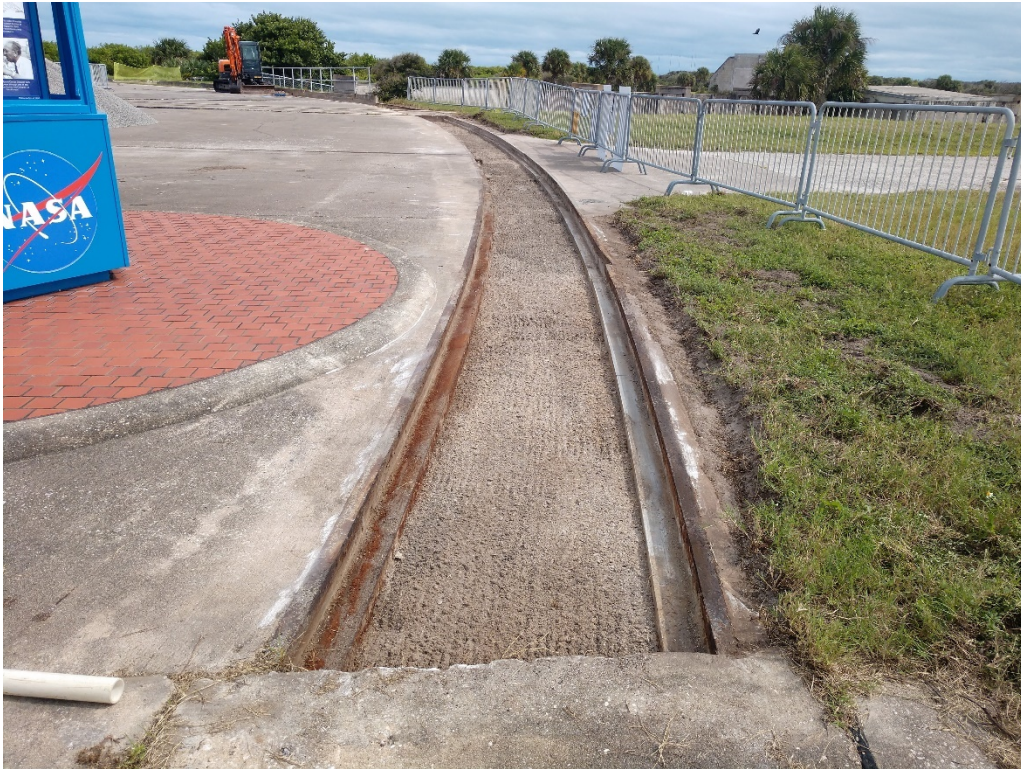
Figure 111: 10/1/2020 3:09:21 PM; facing SE, excavated trench on S side of launch pad
