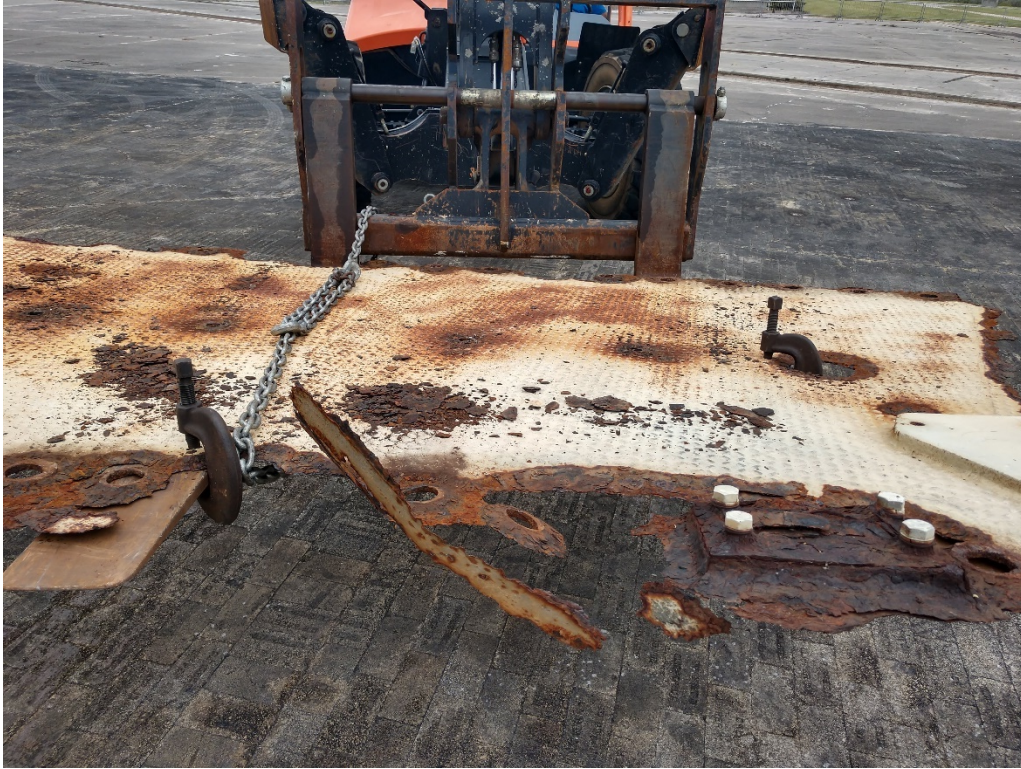
Figure 61: 9/24/2020 11:30:55 AM; top side steel plate removed from Pedestal
