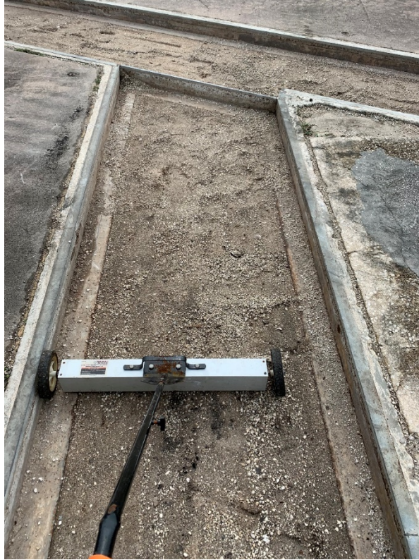
Figure 123: 10/5/2020 3:12:18 PM; removing metal fragments from excavated trench with magnet
