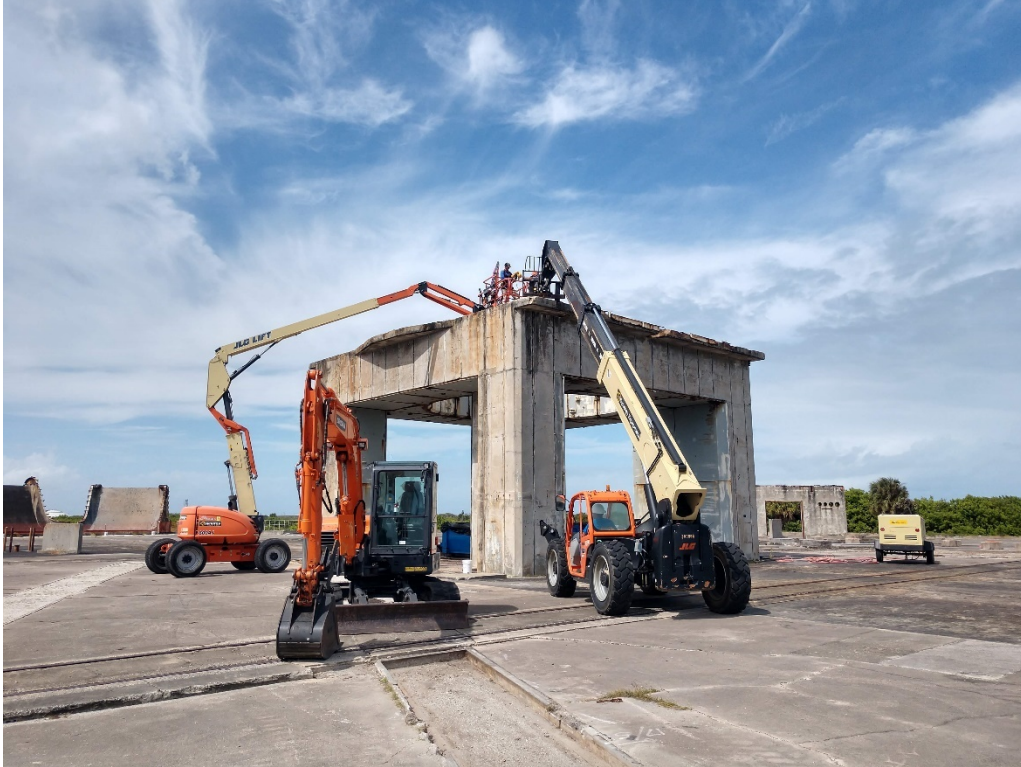
Figure 63: 9/24/2020 2:46:51 PM; removing top side steel plates
