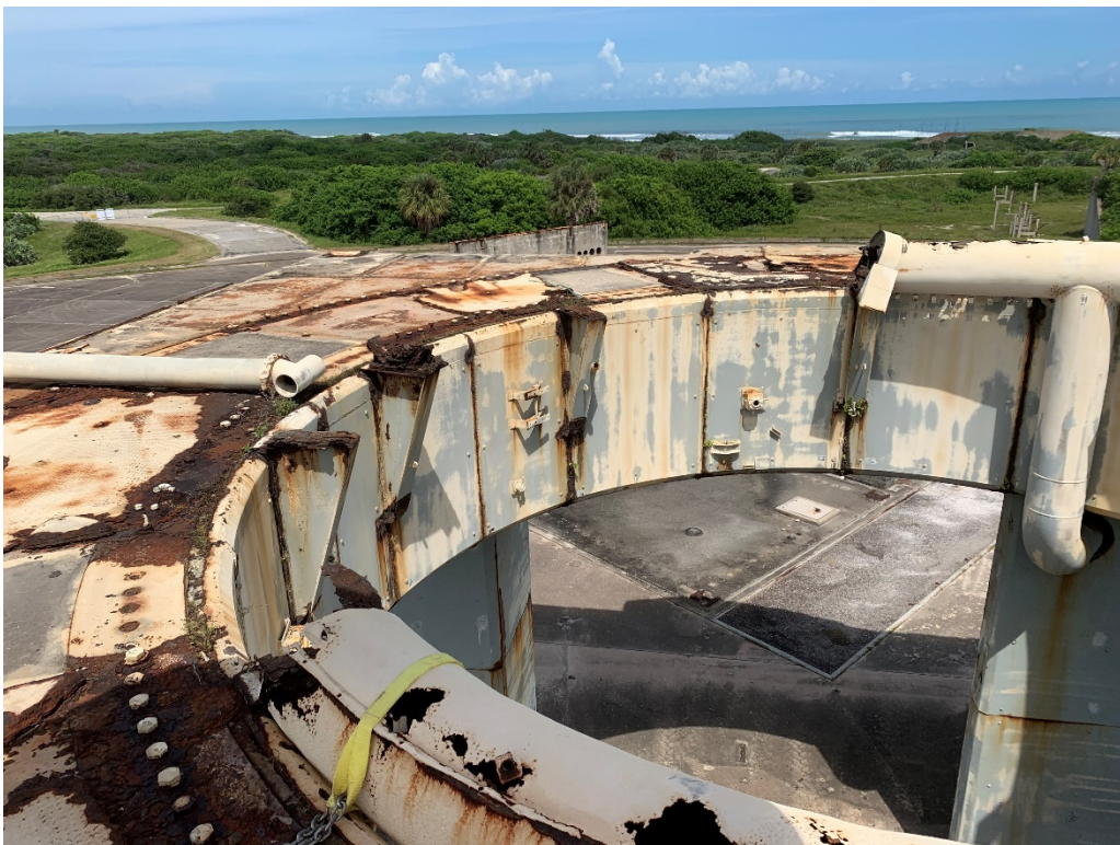
Figure 28: 9/15/2020 2:00:46 PM; top of Pedestal with multiple sections of Torus Ring removed
