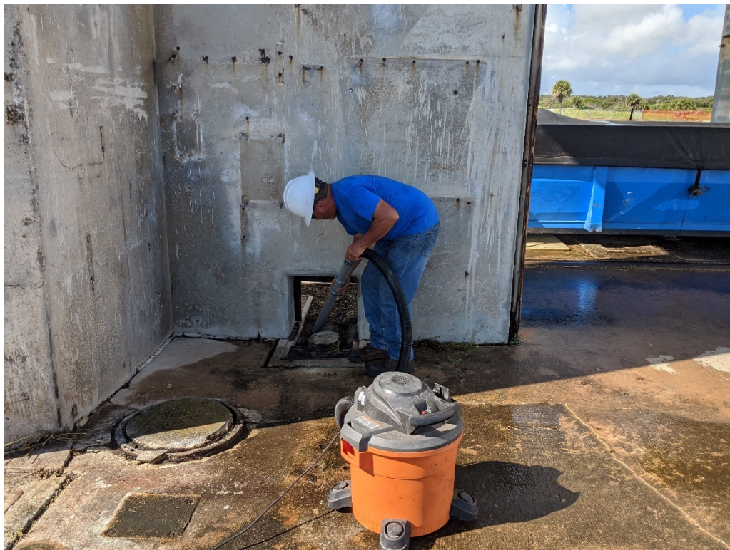
Figure 12: 9/11/2020 10:11:41 AM; vacuuming trench on launch pad near Pedestal
