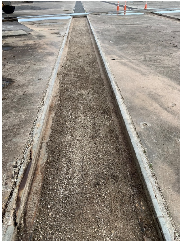
Figure 120: 10/5/2020 3:10:28 PM; facing SE, excavated trench on S side of Pedestal
