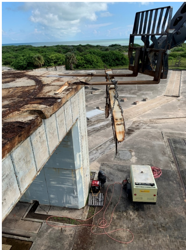
Figure 70: 9/29/2020 10:21:39 AM; lower top side/side edge steel panel
