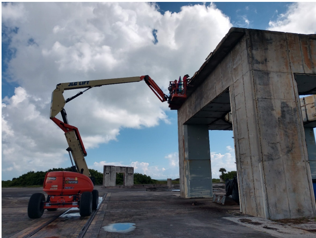
Figure 72: 9/29/2020 11:06:23 AM; removing side edge panels from top of Pedestal
