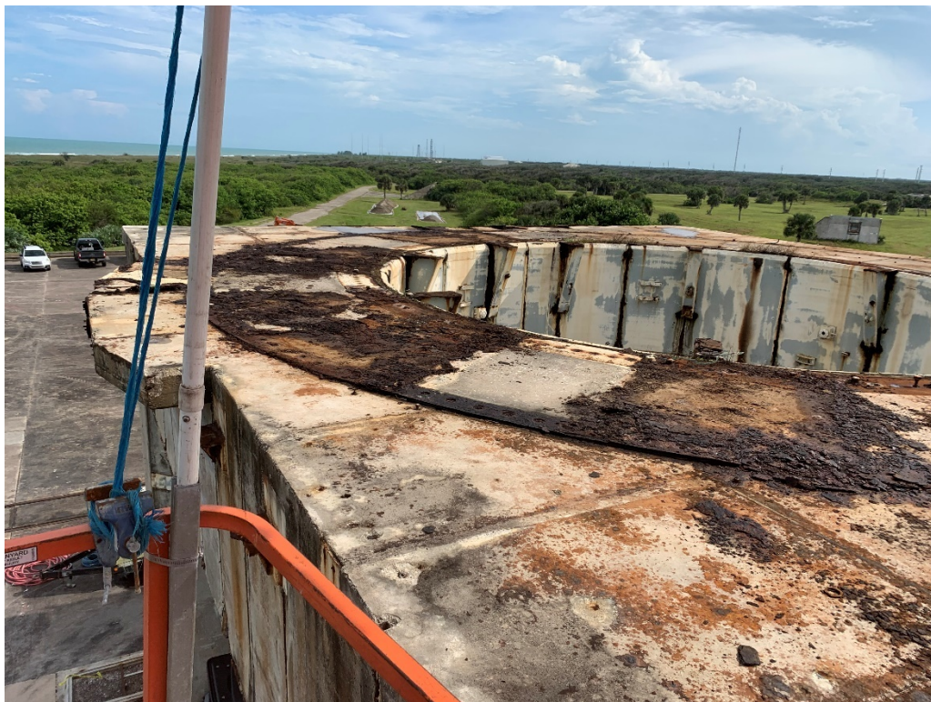
Figure 68: 9/28/2020 3:40:04 PM; top side of Pedestal with steel plates removed
