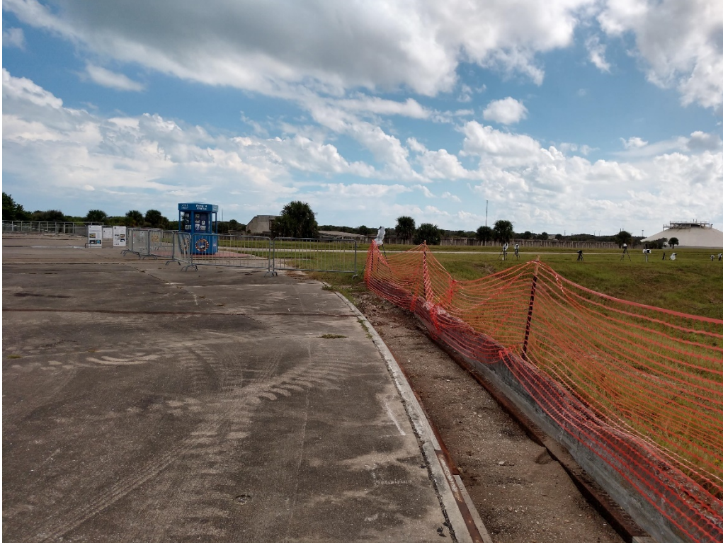
Figure 101: 9/29/2020 3:30:44 PM; facing S, excavated trench on SW side of launch pad
