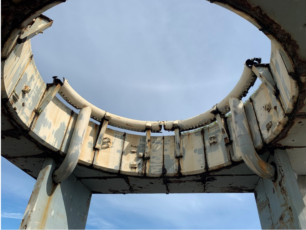
Figure 33: 9/15/2020 3:57:46 PM; looking from underneath Pedestal with sections of Torus Ring removed
