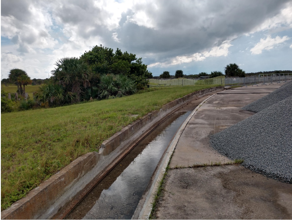
Figure 95: 9/29/2020 3:26:17 PM; facing SW, excavated trench on S side of launch pad
