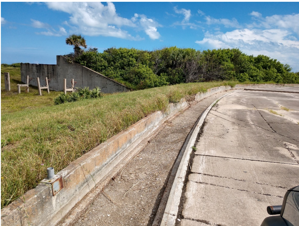
Figure 86: 9/29/2020 3:21:32 PM; facing SE, excavated trench on NE side of launch pad
