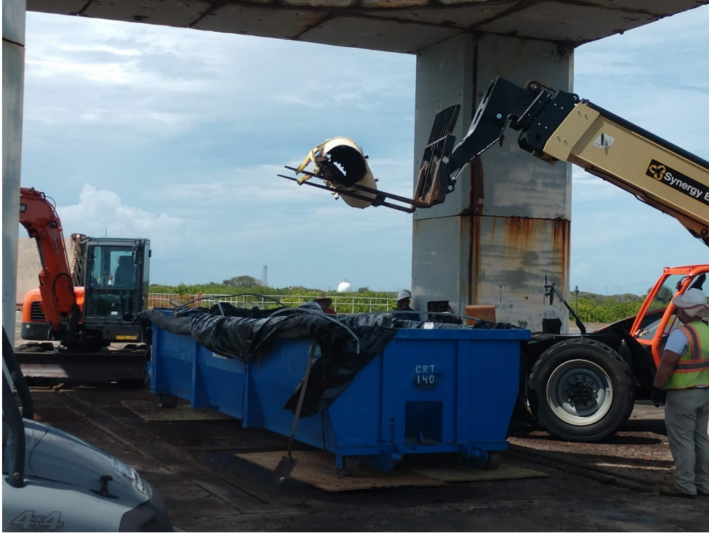
Figure 29: 9/15/2020 2:30:05 PM; lowering section of Torus Ring into roll-off box
