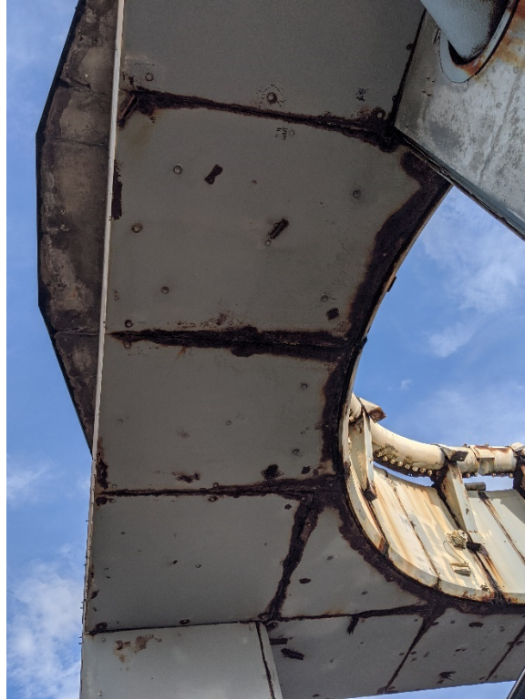
Figure 15: 9/14/2020 9:27:00 AM; looking at underside steel plates with newly installed anchors
