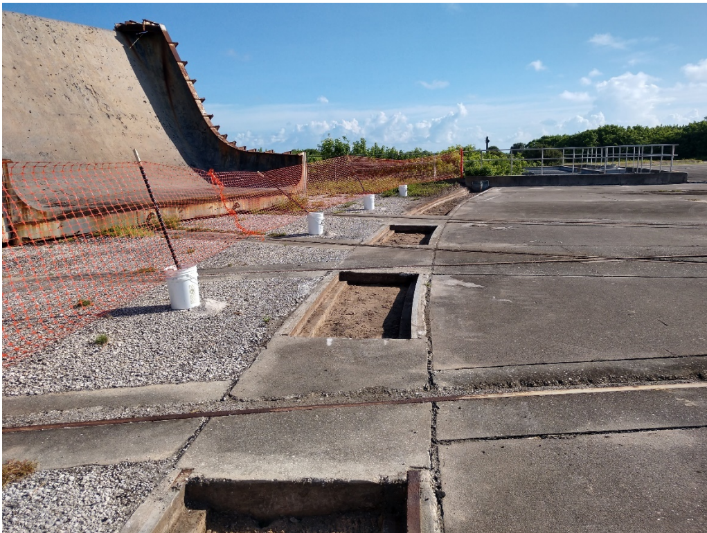
Figure 18: 9/15/2020 9:35:05 AM; facing NE, excavated trenches of NW side of launch pad
