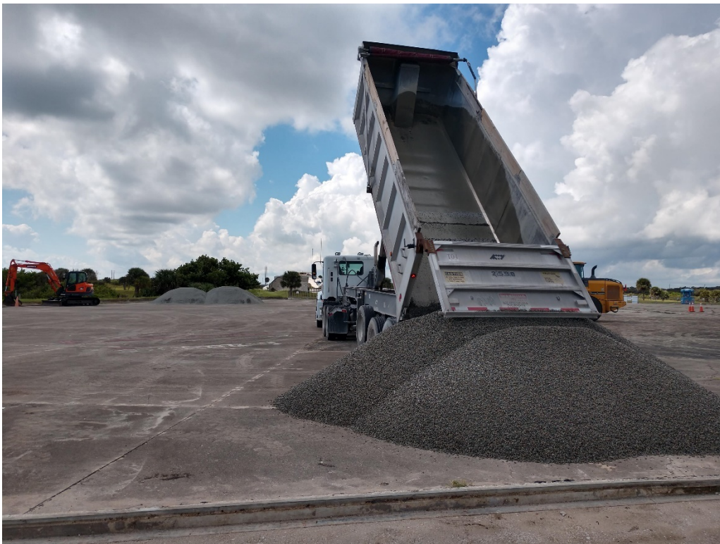
Figure 74: 9/29/2020 11:36:34 AM; granite stone stockpile
