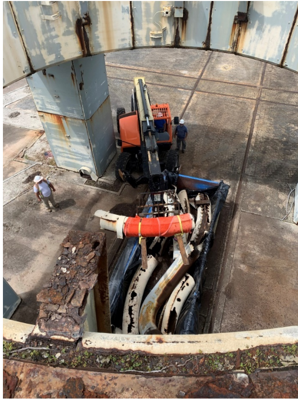
Figure 45: 9/16/2020 1:26:13 PM; removing Torus Ring section into roll-off box
