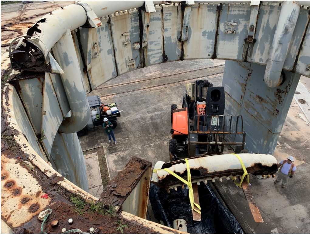
Figure 25: 9/15/2020 11:57:18 AM; lowering section of Torus Ring into roll-off box
