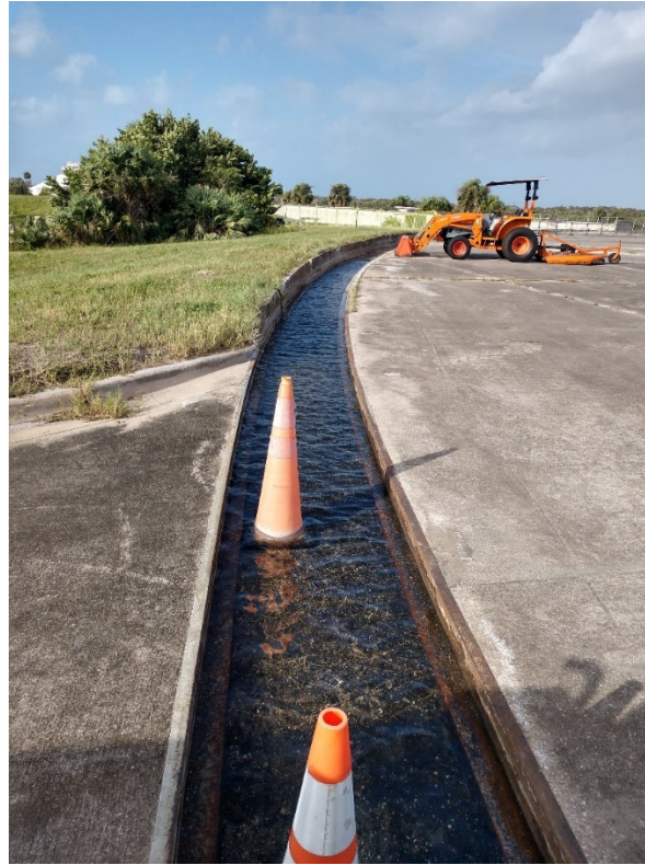
Figure 55: 9/21/2020 9:09:12 AM; facing SW, excavated trench on SE side of launch pad
