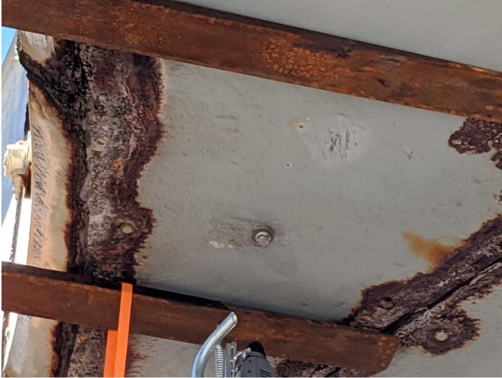
Figure 7: 9/9/2020 1:14:05 PM; newly installed anchor on underside steel plate
