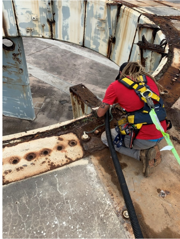
Figure 77: 9/29/2020 3:12:32 PM; vacuuming top of the Pedestal
