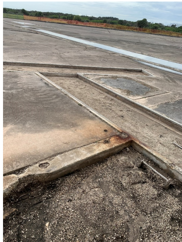
Figure 122: 10/5/2020 3:10:33 PM; facing SW, excavated trenches on SW side of Pedestal
