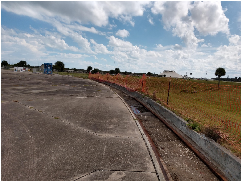
Figure 100: 9/29/2020 3:30:30 PM; facing S, excavated trench on SW side of launch pad
