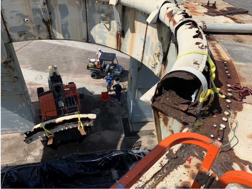
Figure 23: 9/15/2020 11:08:19 AM; lowering section of Torus Ring into roll-off box
