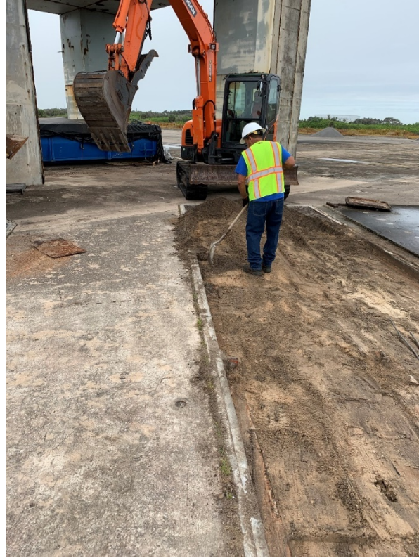
Figure 103: 9/30/2020 10:04:58 AM; facing SW, hand digging trench on NE side of launch pad
