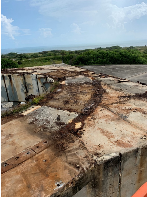
Figure 65: 9/25/2020 10:48:20 AM; top side of Pedestal with steel plates removed
