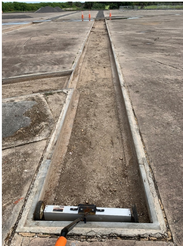
Figure 124: 10/5/2020 3:12:32 PM; removing metal fragments from excavated trench with magnet
