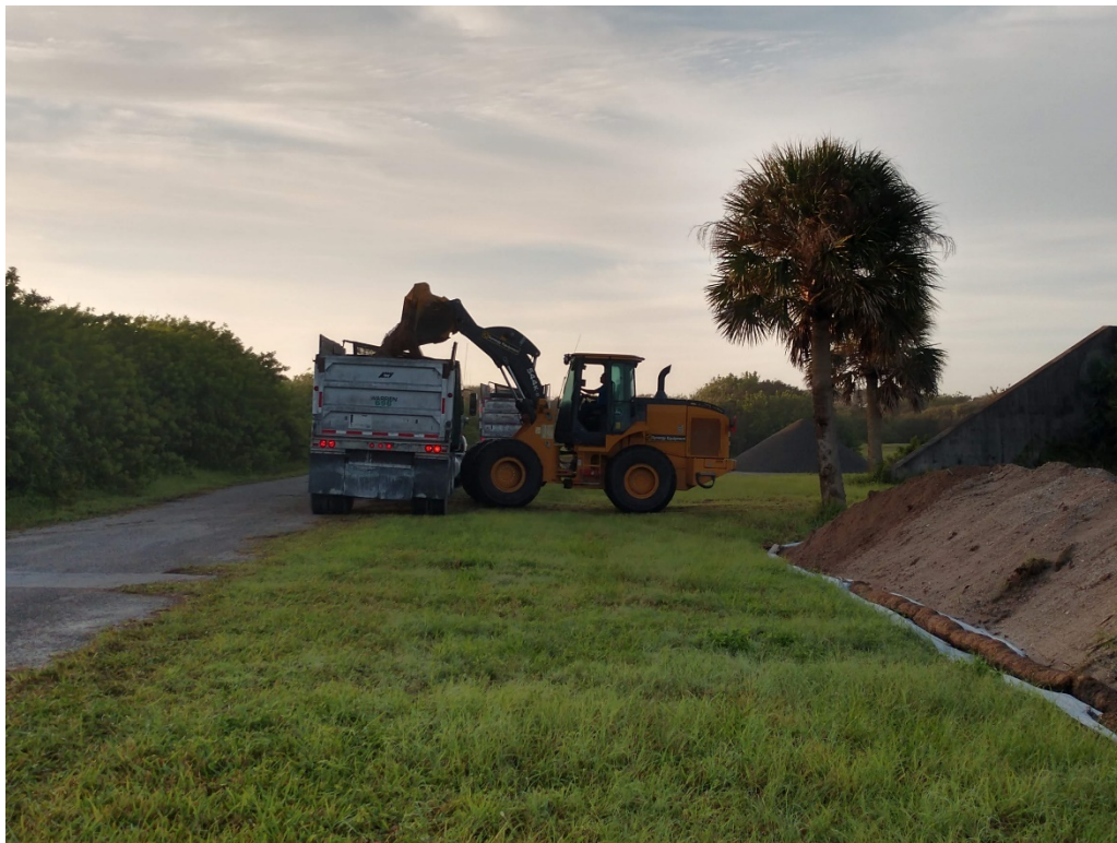
Figure 130: 10/7/2020 7:45:32 AM; excavated soil stockpile being loaded into T&D truck
