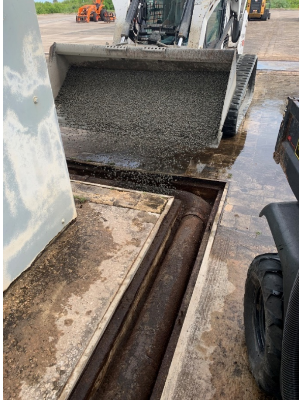
Figure 127: 10/5/2020 3:33:06 PM; backfilling trenches
