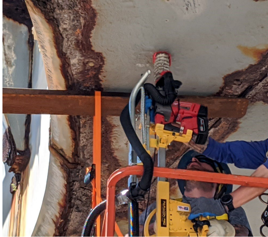
Figure 5: 9/9/2020 1:07:50 PM; drilling hole for anchor installation
