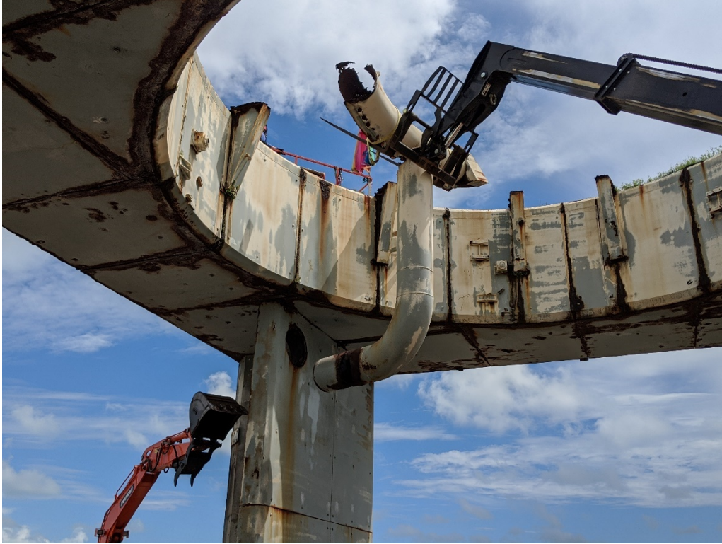
Figure 49: 9/16/2020 1:48:27 PM; lowering Torus Ring section and down pipe
