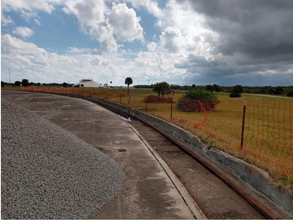
Figure 99: 9/29/2020 3:29:59 PM; facing S, excavated trench on W side of launch pad
