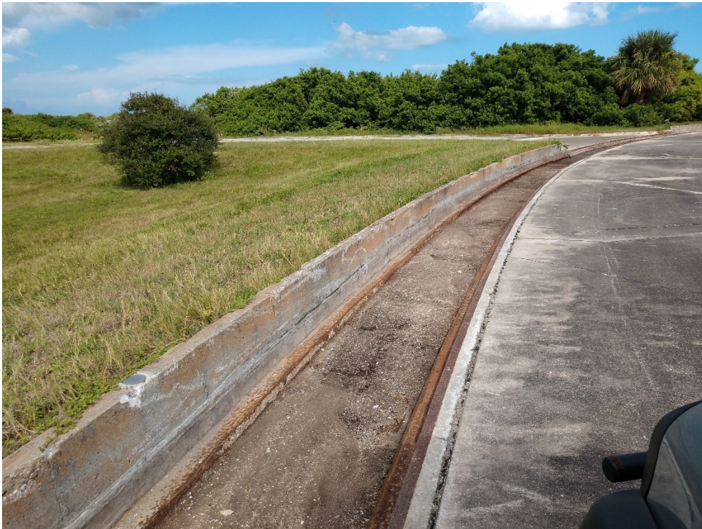
Figure 82: 9/29/2020 3:20:34 PM; facing N, excavated trench on NW side of launch pad
