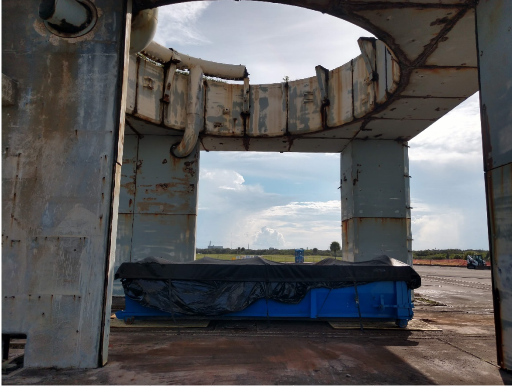
Figure 37: 9/15/2020 4:28:48 PM; looking from underneath Pedestal with sections of Torus Ring removed
