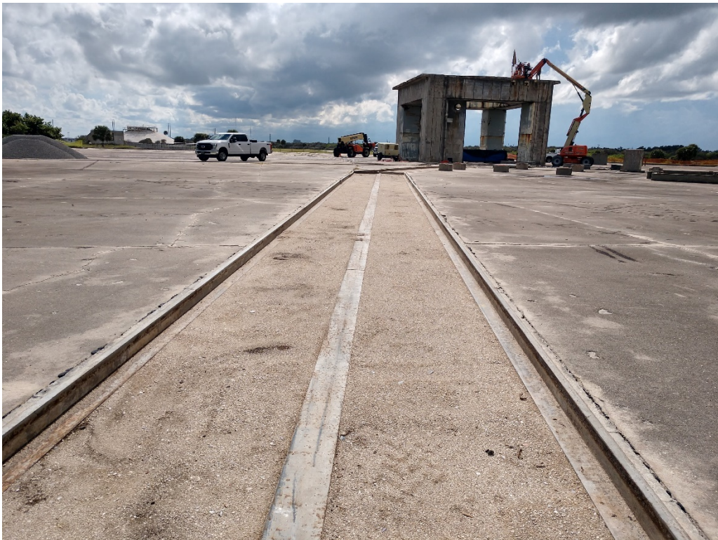
Figure 88: 9/29/2020 3:22:12 PM; facing SW, excavated trench on NE side of launch pad
