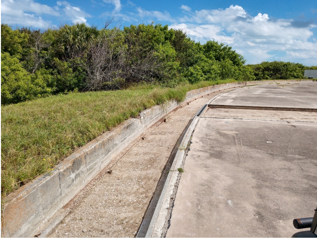
Figure 87: 9/29/2020 3:21:46 PM; facing SE, excavated trench on NE side of launch pad
