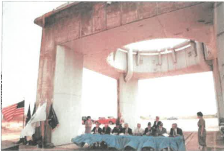
Figure 7. The Launch Pedestal following restoration activities in the 1990s
