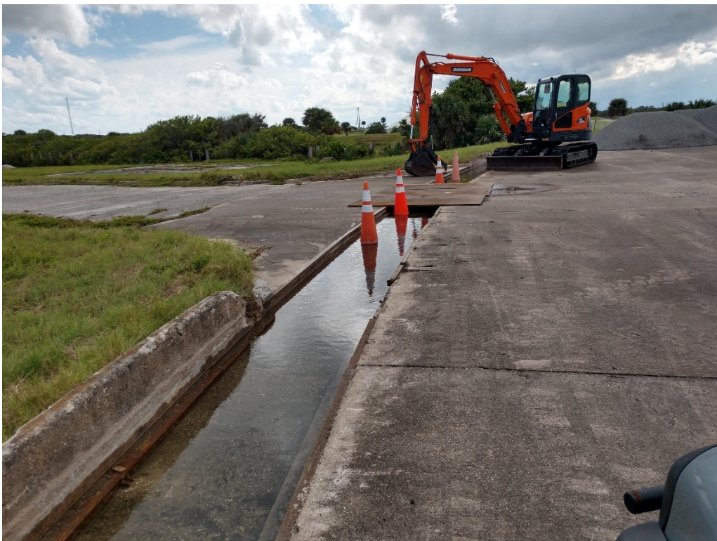
Figure 94: 9/29/2020 3:25:58 PM; facing S, excavated trench on SE side of launch pad
