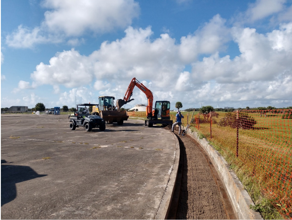
Figure 21: 9/15/2020 9:36:57 AM; facing S, excavated trenches on W side of launch pad
