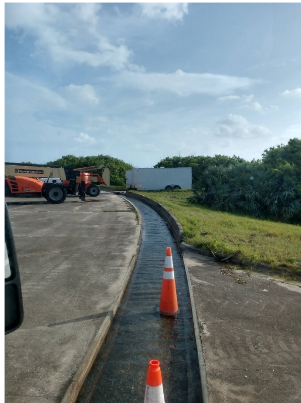
Figure 56: 9/21/2020 9:09:23 AM; facing NW, excavated trench on SE side of launch pad
