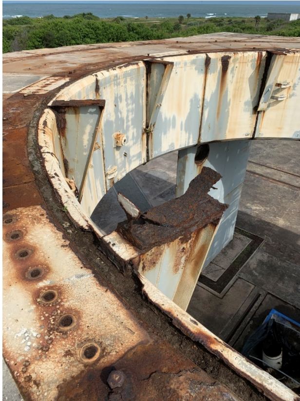
Figure 105: 9/30/2020 3:32:07 PM; top of the Pedestal after sweeping and vacuuming
