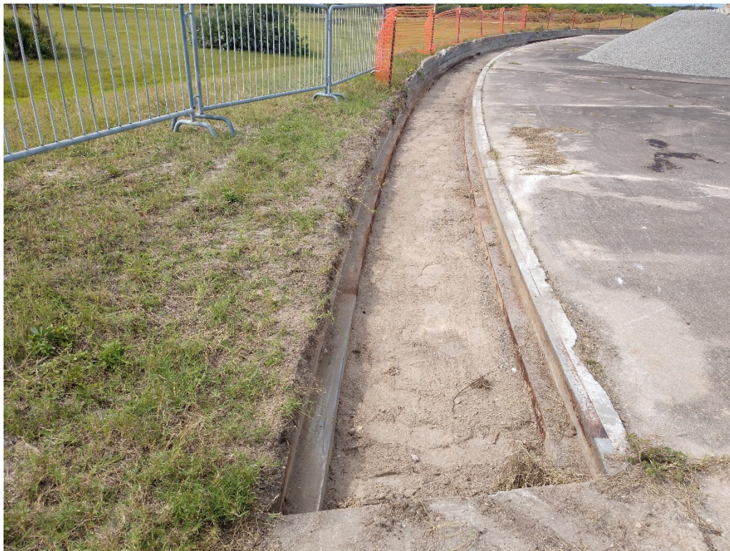
Figure 110: 10/1/2020 3:09:12 PM; facing W, excavated trench of SW side of launch pad
