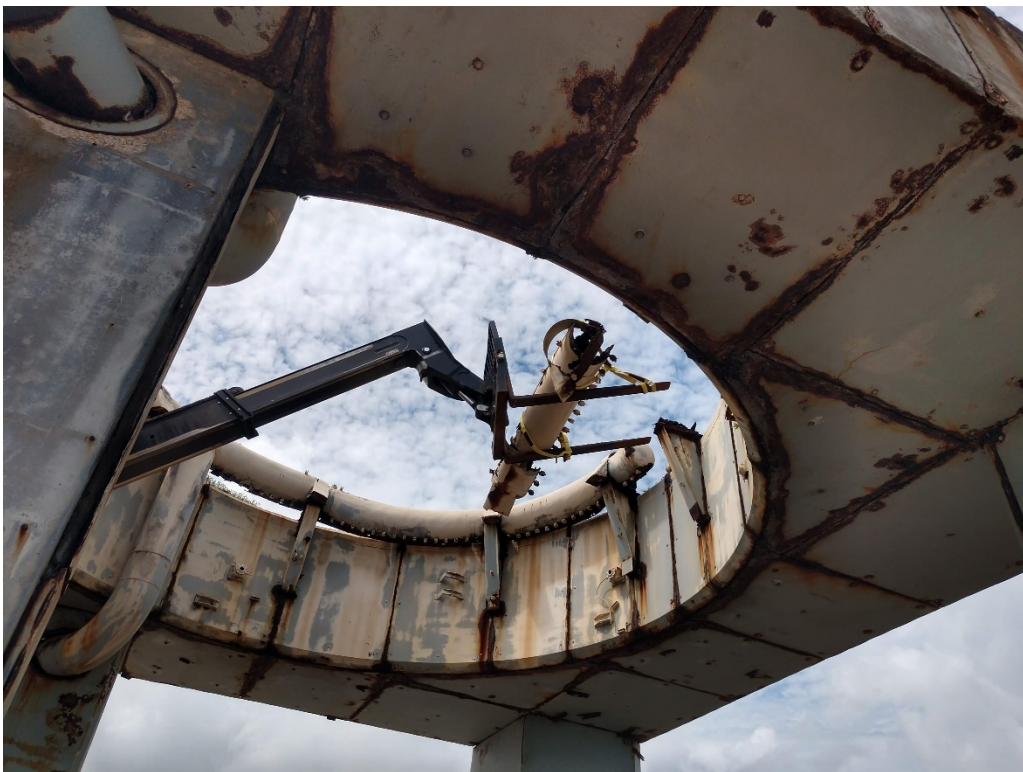
Figure 24: 9/15/2020 11:57:01 AM; lowering section of Torus Ring into roll-off box
