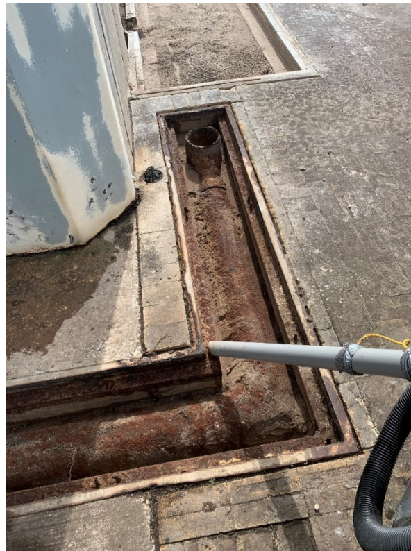
Figure 128: 10/5/2020 3:41:10 PM; facing SE, vacuuming trench S of Pedestal
