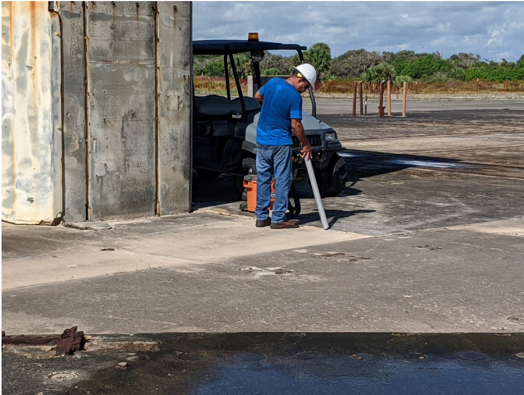
Figure 9: 9/10/2020 10:32:18 AM; vacuuming steel fragments from launch pad
