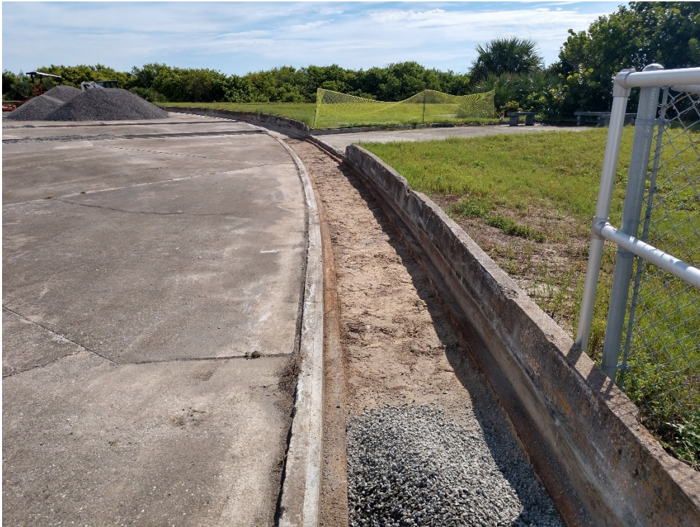
Figure 117: 10/2/2020 11:01:45 AM; facing E, backfilling trench on S side of launch pad
