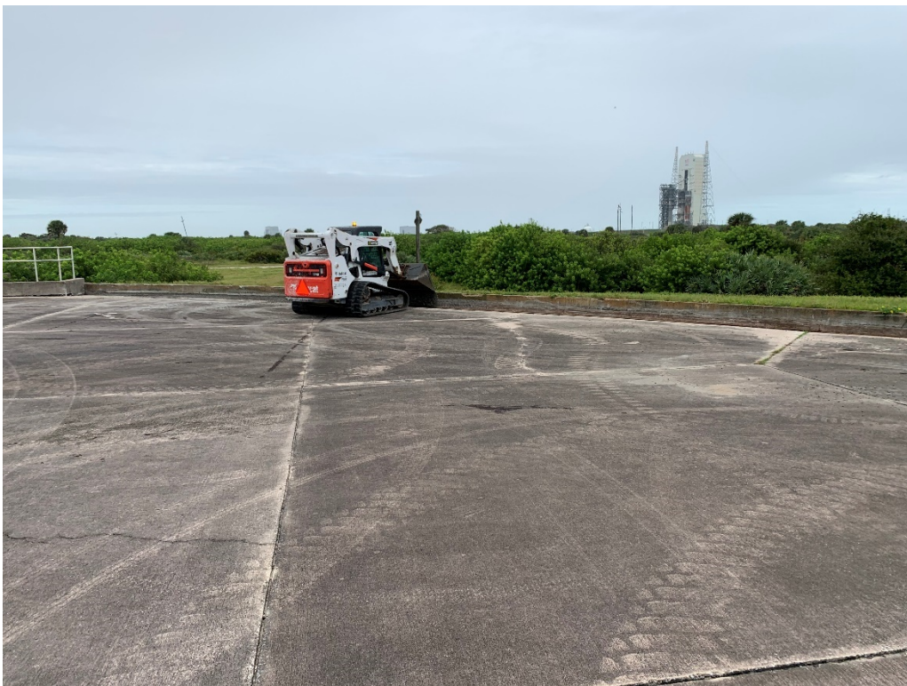
Figure 102: 9/30/2020 10:02:52 AM; backfilling on N side of launch pad
