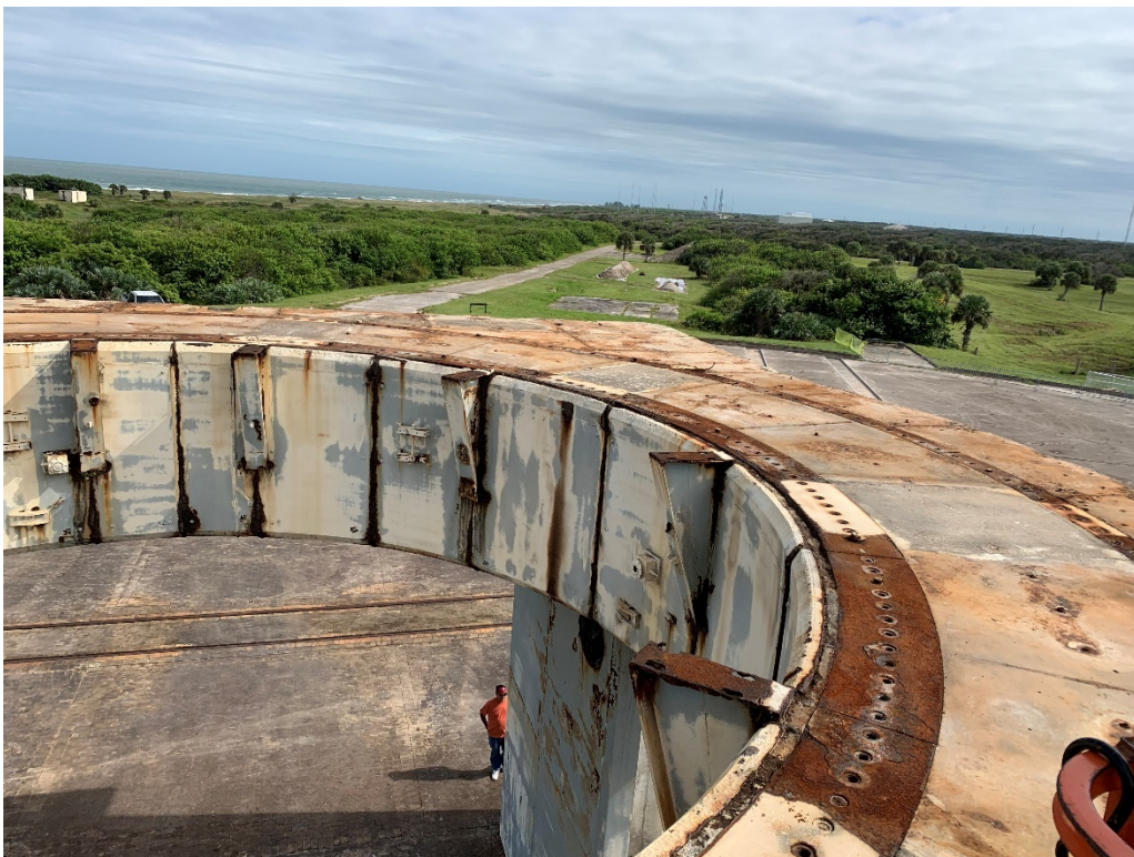
Figure 108: 9/30/2020 3:32:16 PM; top of the Pedestal after sweeping and vacuuming
