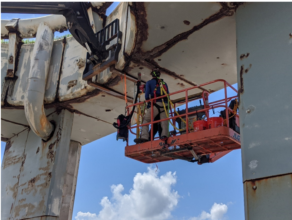
Figure 10: 9/10/2020 11:55:30 AM; drilling hole for anchor installation
