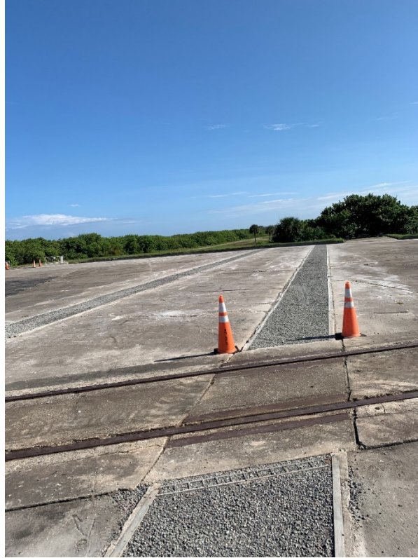
Figure 133: 10/8/2020 3:35:54 PM; facing SE, launch pad following restoration activities
