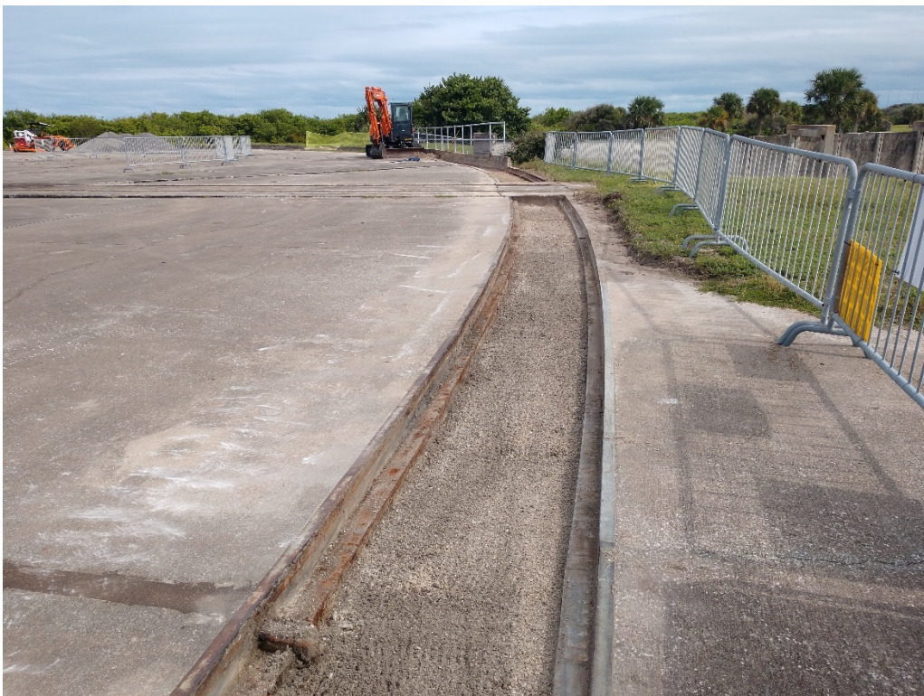
Figure 112: 10/1/2020 3:09:40 PM; facing SE, excavated trench on S side of launch pad
