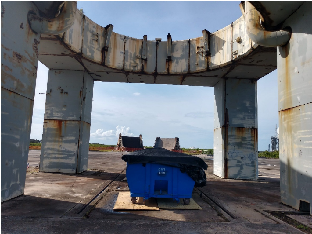
Figure 34: 9/15/2020 4:26:54 PM; looking from underneath Pedestal with sections of Torus Ring removed
