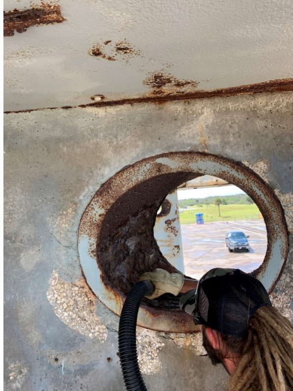
Figure 75: 9/29/2020 1:45:09 PM; vacuuming debris from down pipe opening
