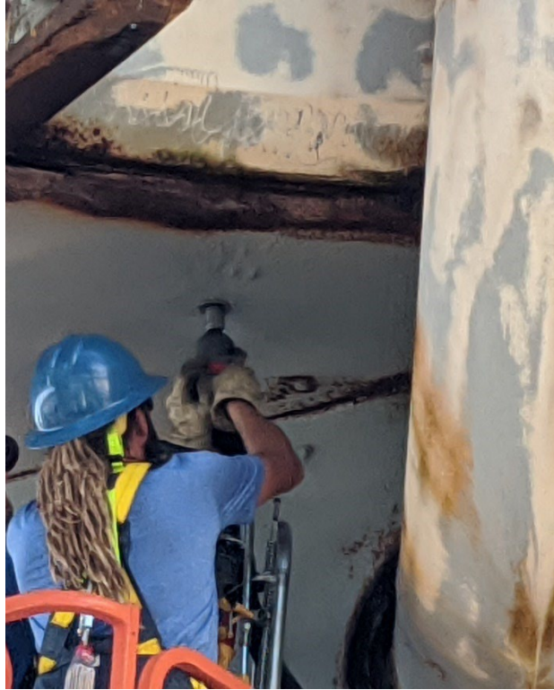
Figure 11: 9/11/2020 10:11:15 AM; drilling hole for anchor installation
