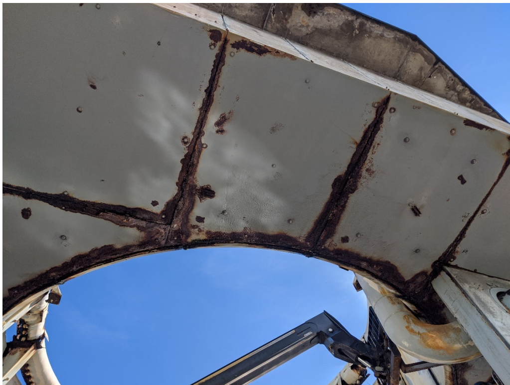
Figure 14: 9/11/2020 10:14:39 AM; looking at underside steel plates with newly installed anchors
