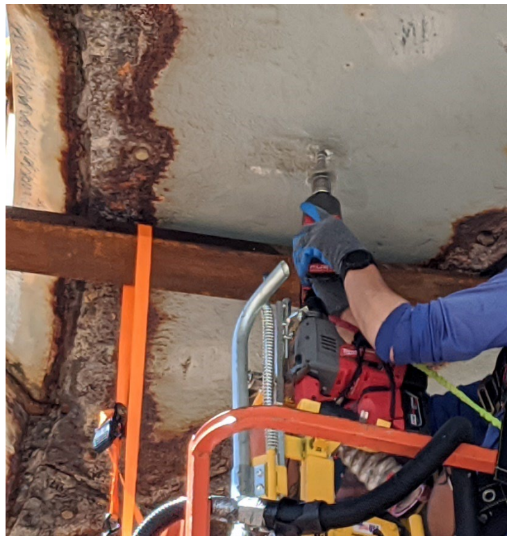
Figure 6: 9/9/2020 1:12:34 PM; anchor installation
