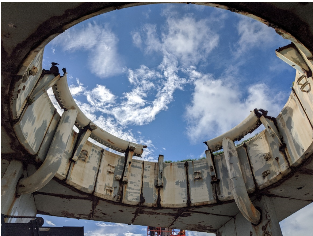
Figure 38: 9/16/2020 9:46:14 AM; looking from underneath Pedestal with sections of Torus Ring removed
