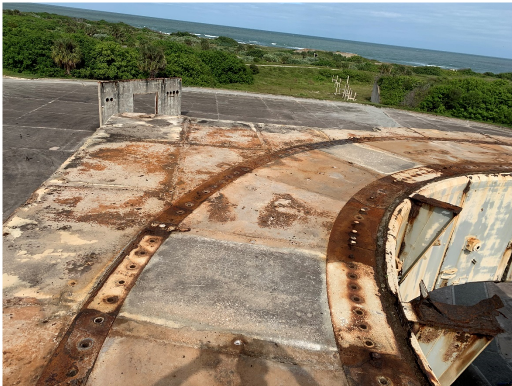
Figure 106: 9/30/2020 3:32:13 PM; top of the Pedestal after sweeping and vacuuming
