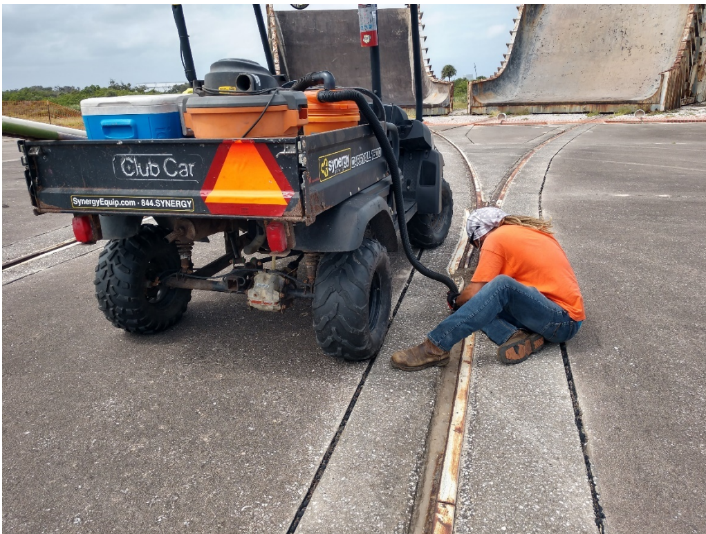
Figure 58: 9/22/2020 1:39:03 PM; facing NW, vacuuming launch pad
