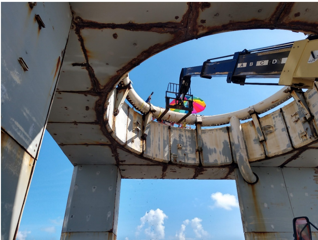
Figure 22: 9/15/2020 10:48:11 AM; securing section of Torus Ring to telehandler
