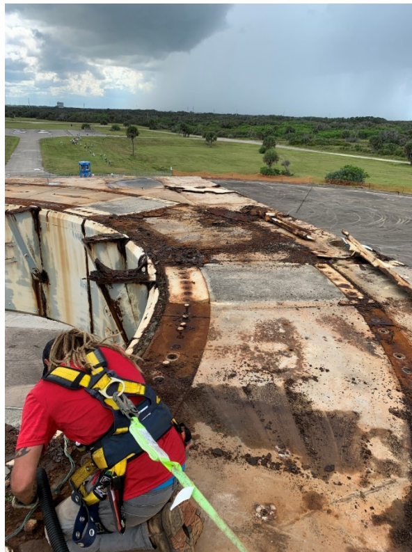
Figure 80: 9/29/2020 3:12:39 PM; vacuuming top of the Pedestal
