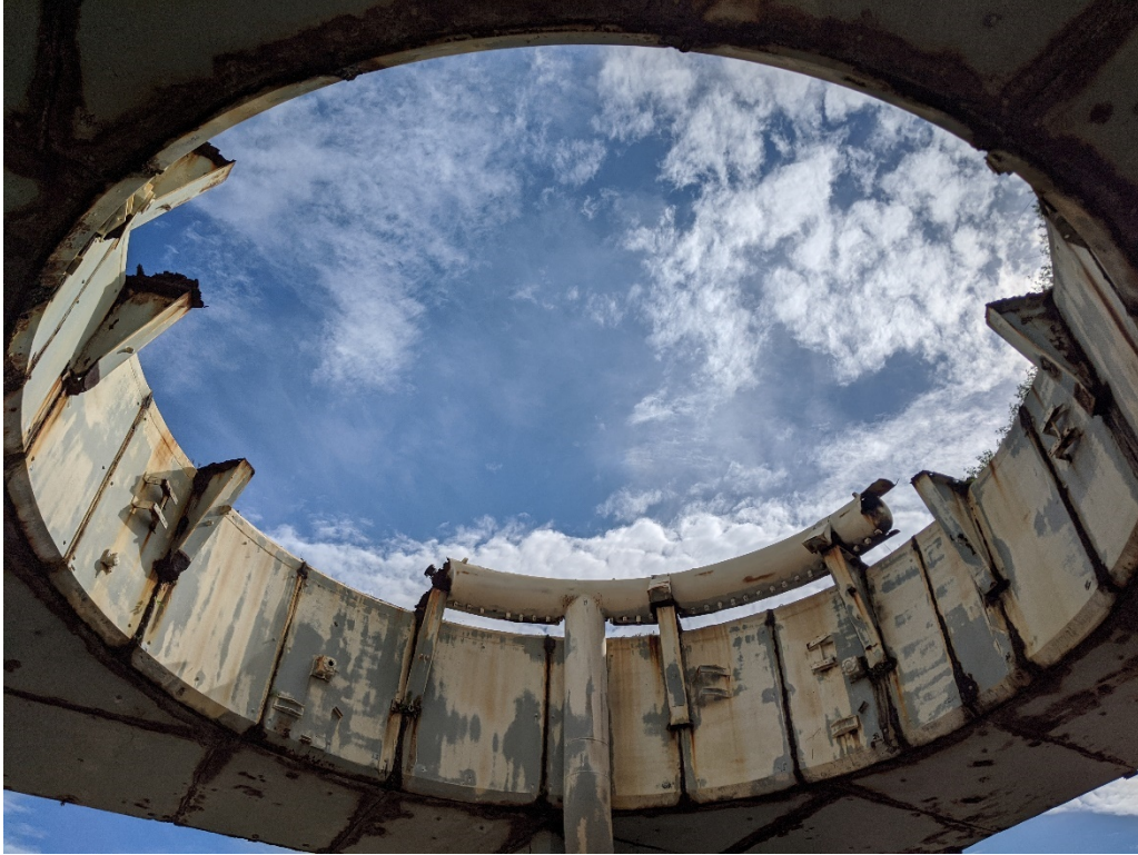
Figure 43: 9/16/2020 10:35:11 AM; Torus Ring section and down pipe to be removed
