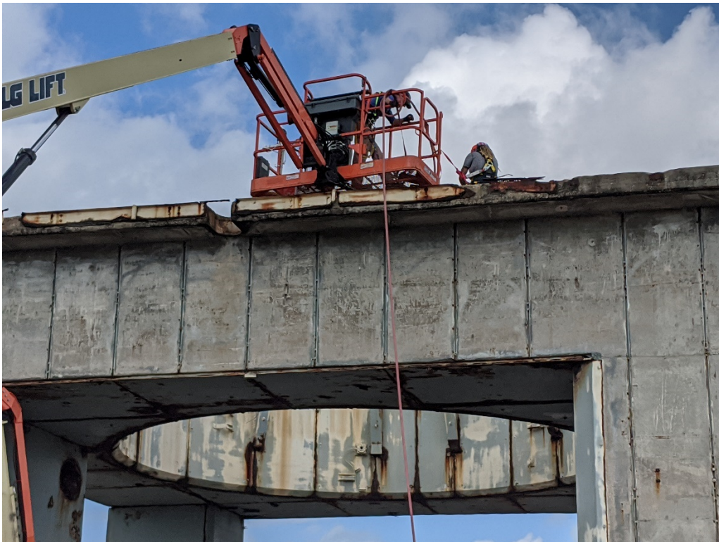
Figure 54: 9/18/2020 11:14:53 AM; removing steel plates from top side of Pedestal
