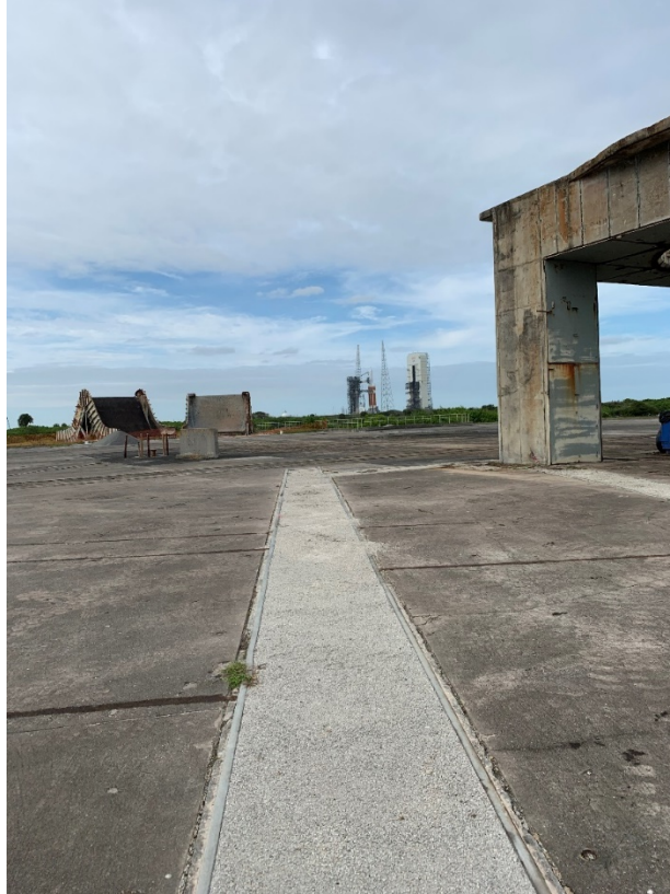
Figure 109: 9/30/2020 4:07:57 PM; facing NW, backfilled trench on S side of launch pad
