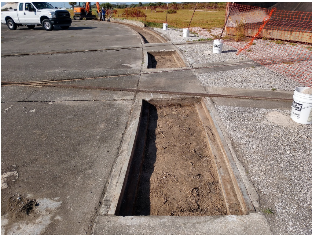
Figure 20: 9/15/2020 9:36:34 AM; facing SW, excavated trenches on NW side of launch pad
