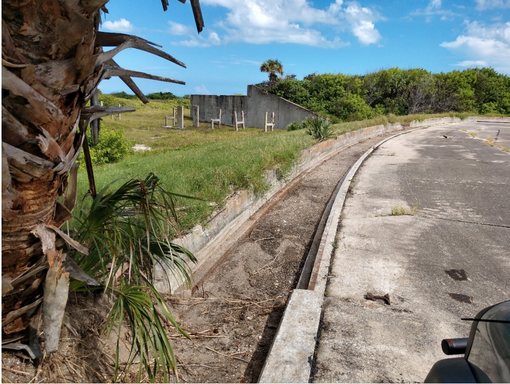
Figure 85: 9/29/2020 3:21:17 PM; facing E, excavated trench on N side of launch pad
