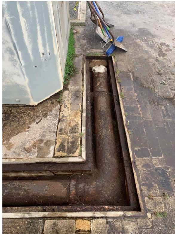
Figure 126: 10/5/2020 3:31:48 PM facing N, vacuumed trench E of Pedestal
