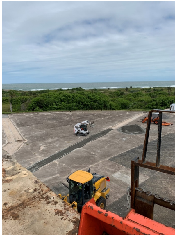
Figure 104: 9/30/2020 1:48:56 PM; facing E, backfilling trench on E side of launch pad
