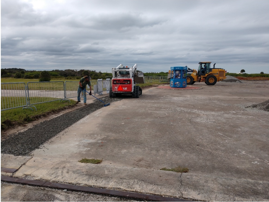
Figure 115: 10/1/2020 3:32:20 PM; facing W, backfilled trench on SW side of launch pad
