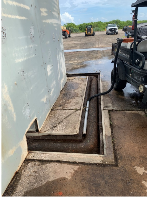
Figure 125: 10/5/2020 3:31:39 PM; facing SE, vacuuming trench S of Pedestal
