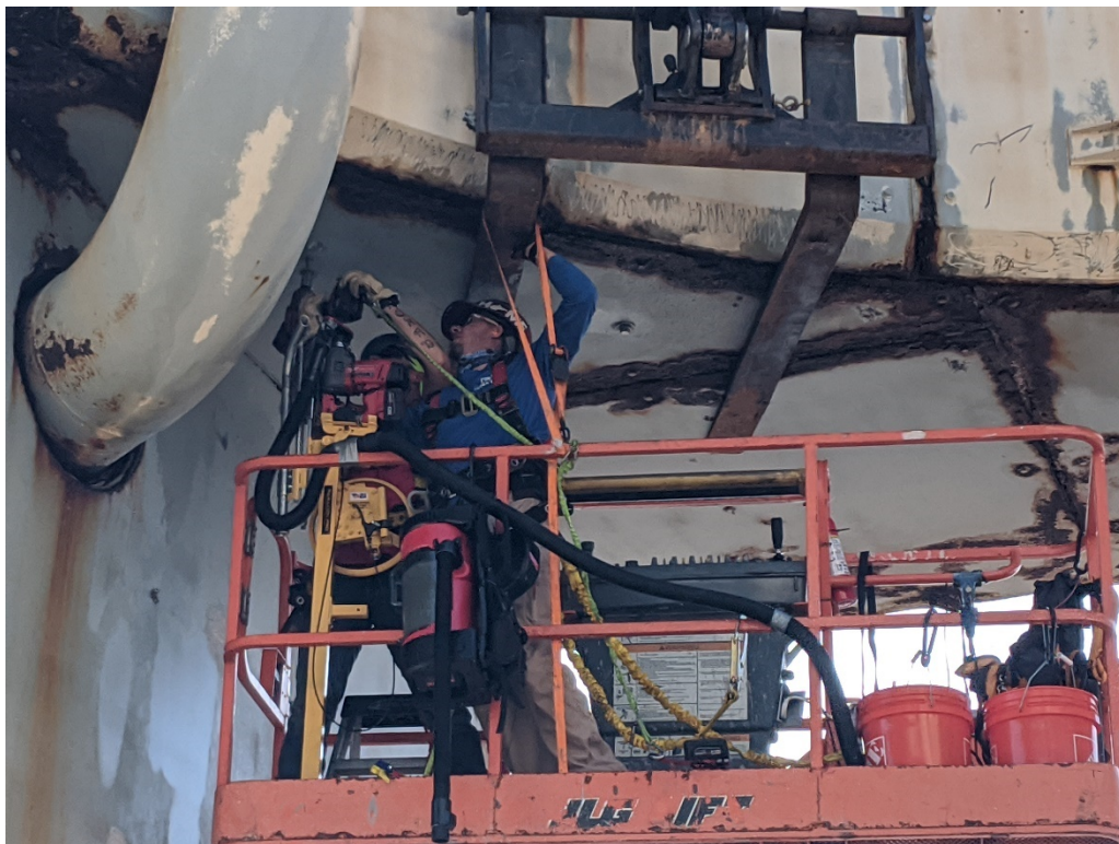
Figure 16: 9/14/2020 10:16:35 AM; drilling hole for anchor installation
