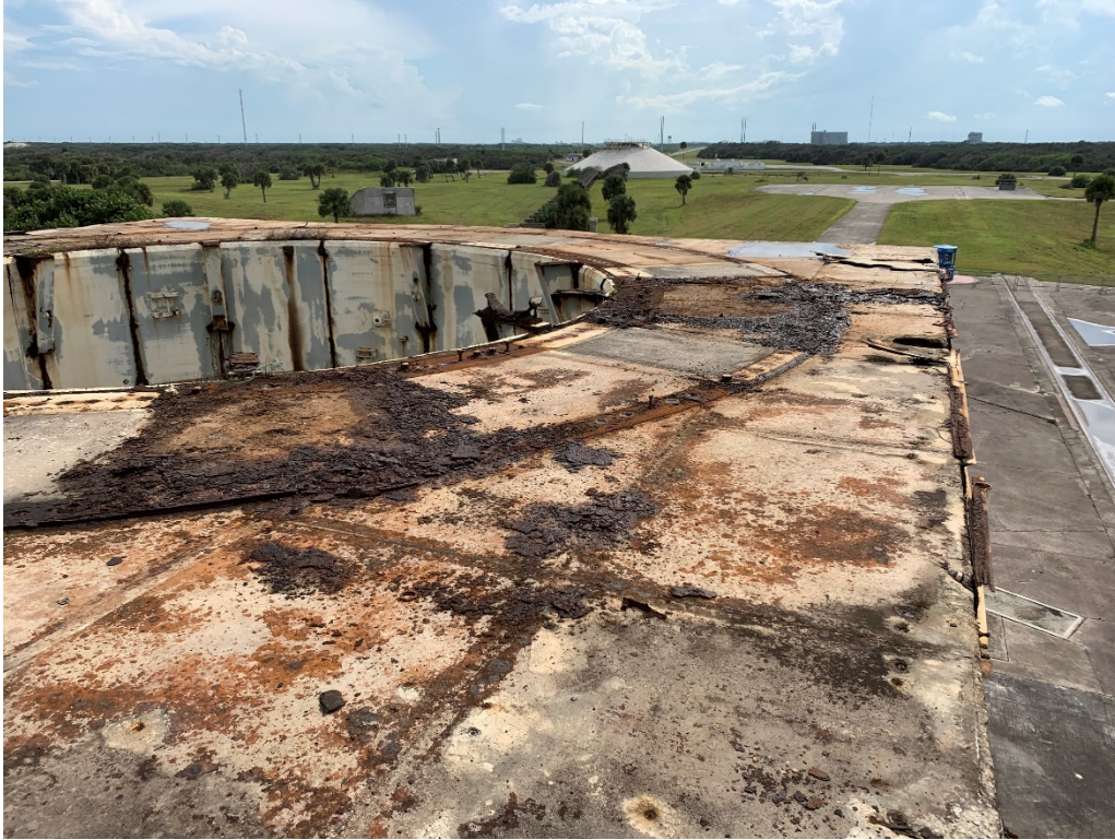
Figure 69: 9/28/2020 3:40:06 PM; top side of Pedestal with steel plates removed
