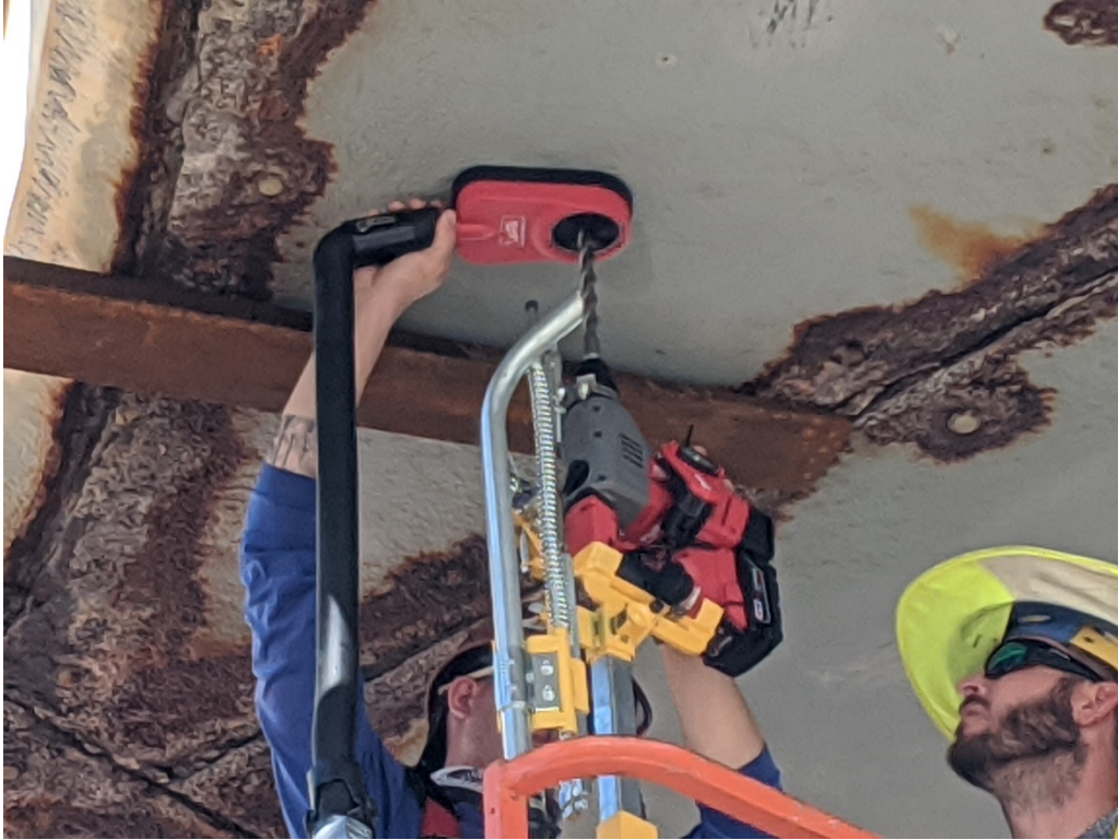
Figure 3: 9/9/2020 10:19:06 AM; drilling hole for anchor installation
