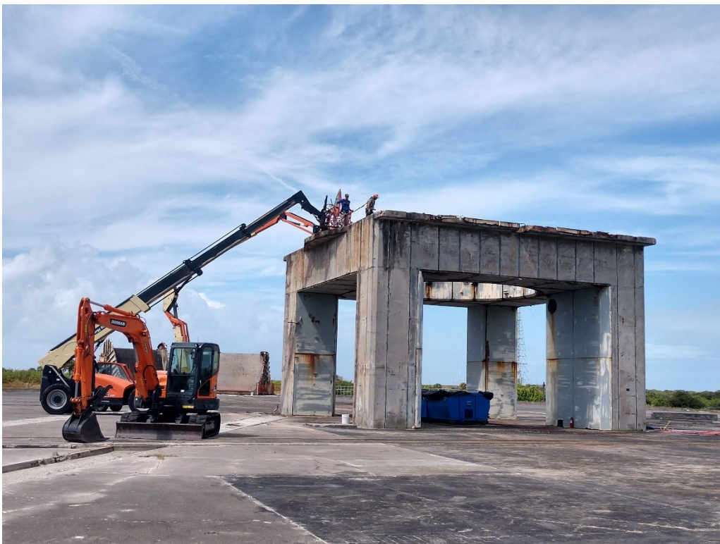
Figure 62: 9/24/2020 2:02:30 PM; removing top side steel plates
