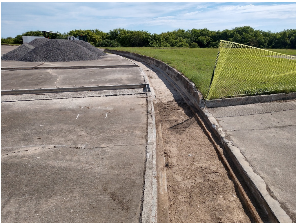
Figure 118: 10/2/2020 11:02:02 AM; facing NE, excavated trench on SE side of launch pad
