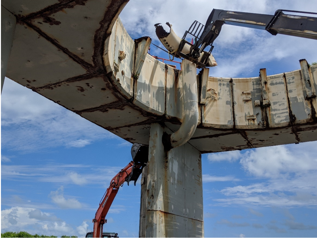
Figure 47: 9/16/2020 1:48:05 PM; removing Torus Ring section and down pipe
