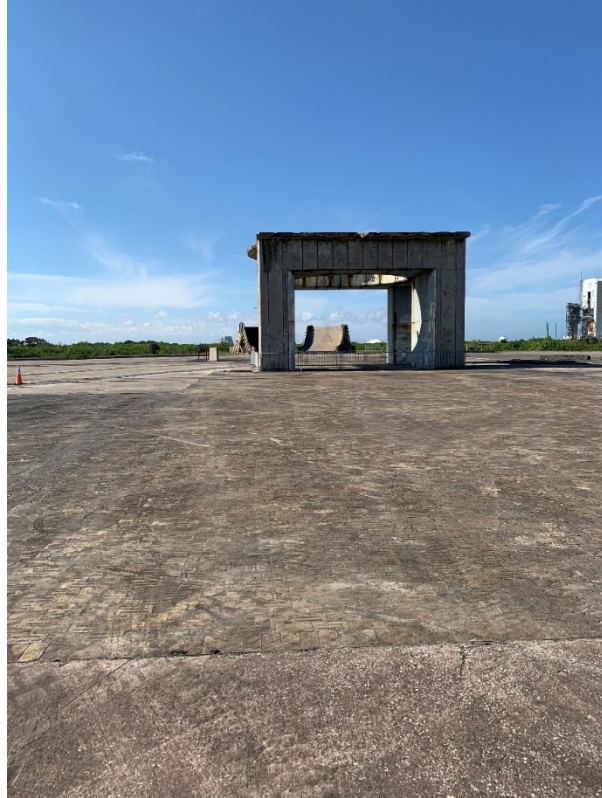
Figure 131: 10/8/2020 3:34:45 PM; facing NW; launch pad and Pedestal following restoration activities
