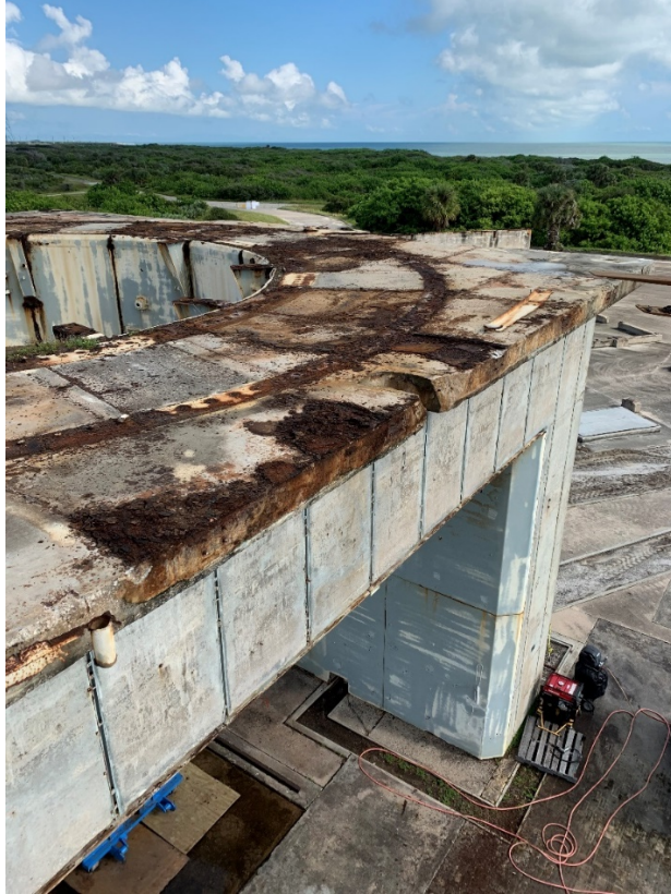
Figure 71: 9/29/2020 10:21:42 AM; top side of Pedestal with steel plates removed
