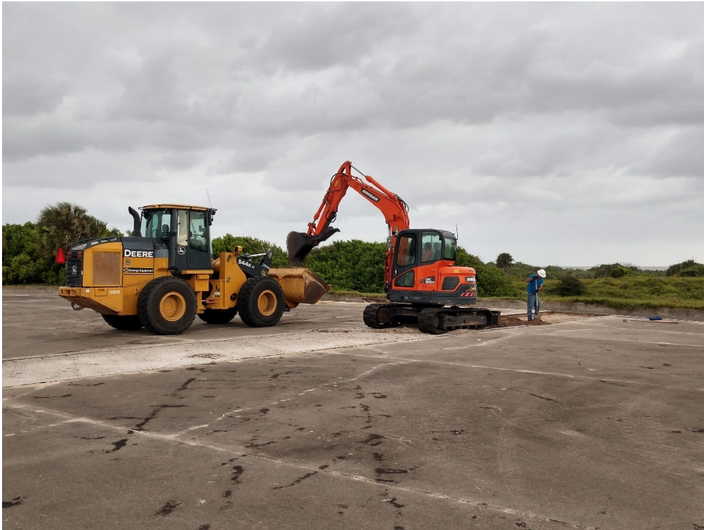
Figure 57: 9/22/2020 8:13:47 AM; facing N, excavating trench on NW side of launch pad
