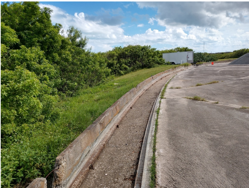
Figure 90: 9/29/2020 3:23:20 PM; facing S, excavated trench on E side of launch pad
