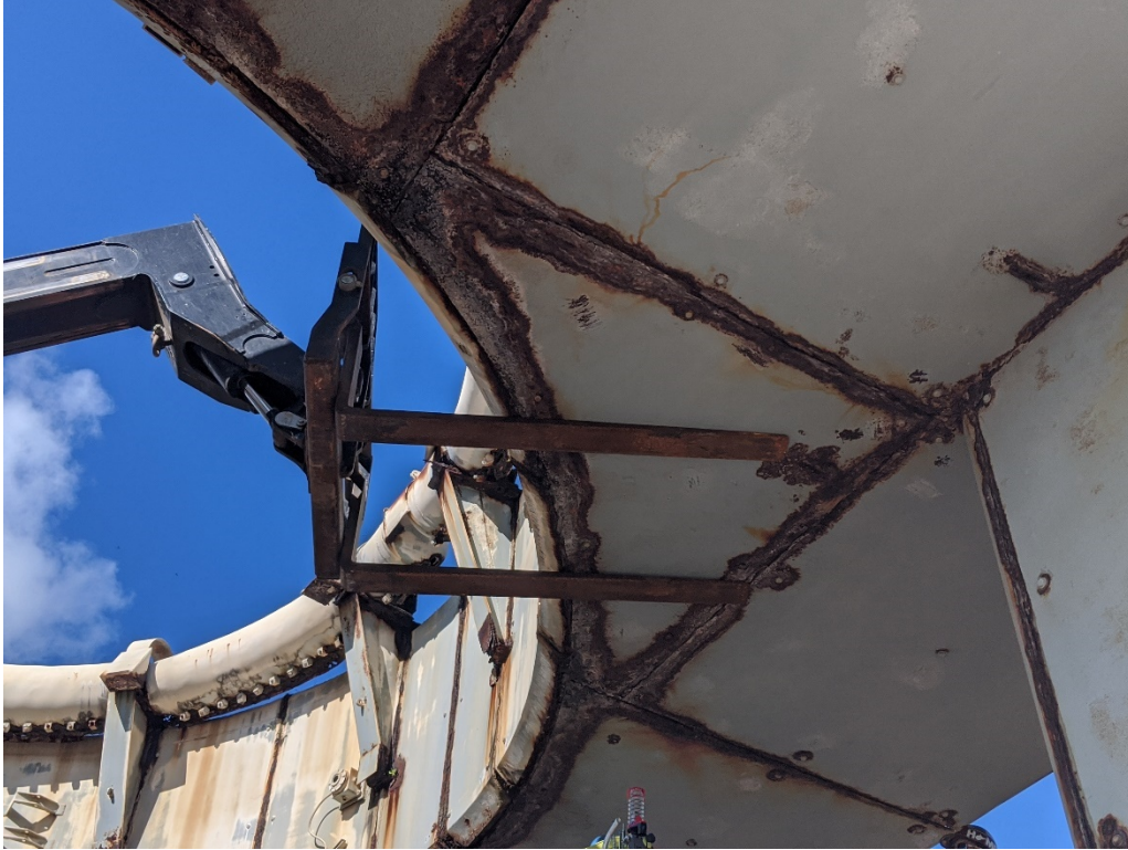
Figure 1: 9/9/2020 9:58:08 AM; Bracing underside steel plate for anchor installation
