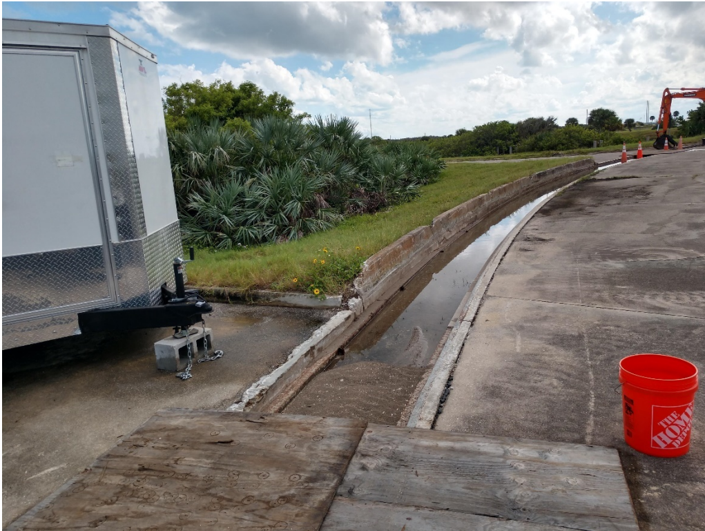
Figure 93: 9/29/2020 3:25:40 PM; facing S, excavated trench on SE side of launch pad
