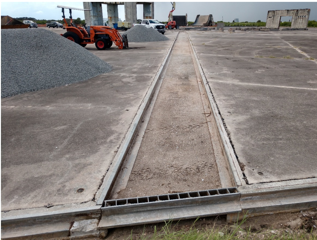
Figure 92: 9/29/2020 3:25:23 PM; facing NW, excavated trench on E side of launch pad
