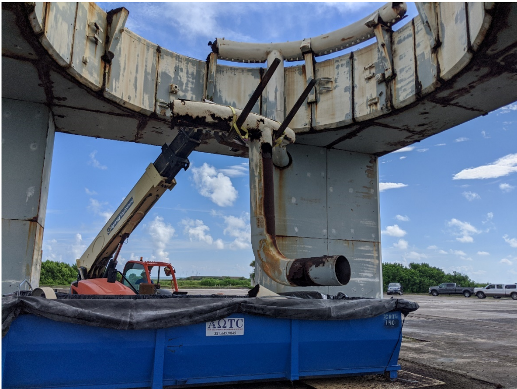
Figure 42: 9/16/2020 10:19:45 AM; lowering Torus Ring section and down pipe
