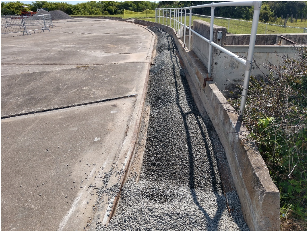
Figure 116: 10/2/2020 11:01:24 AM; facing E, backfilling trench on S side of launch pad
