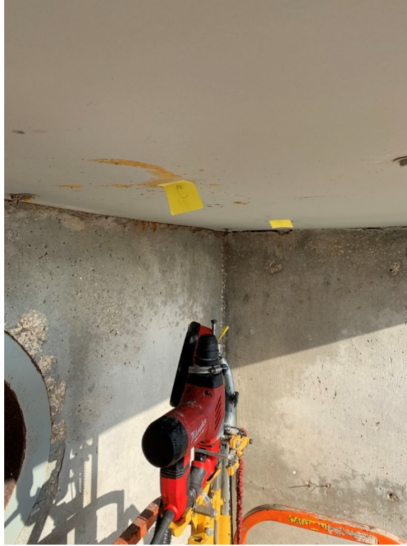
Figure 137: 11/16/2020 3:37:57 PM; marked anchor locations of "phase 2"
