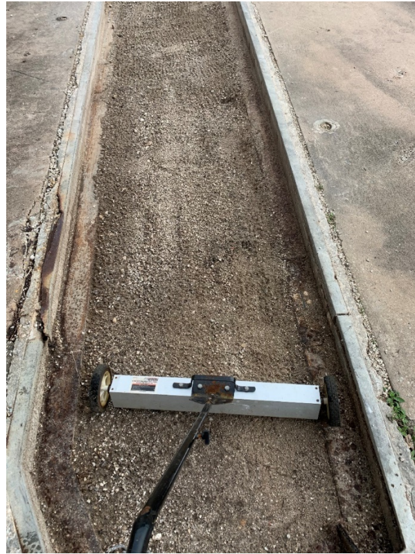
Figure 121: 10/5/2020 3:10:30 PM; removing metal debris from excavated trench with magnet
