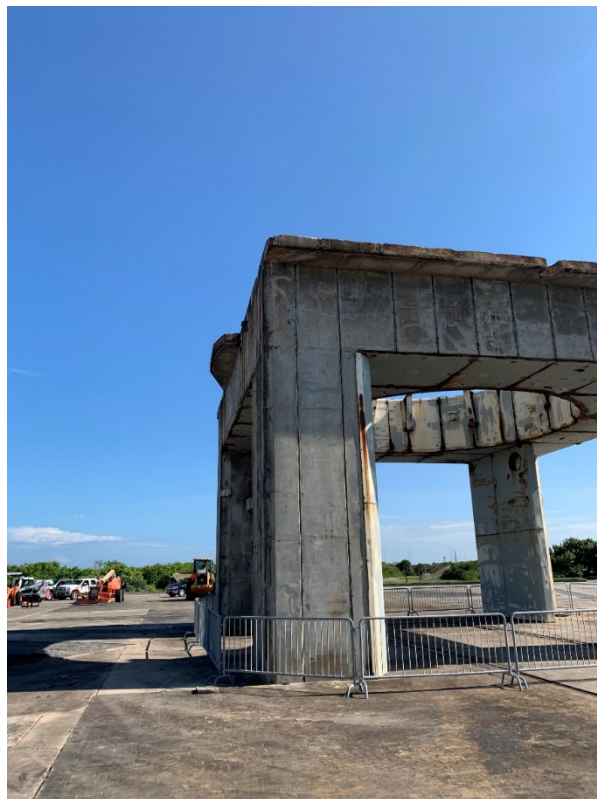
Figure 134: 10/8/2020 3:36:55 PM; facing SE, Pedestal following restoration activities
