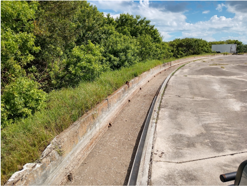
Figure 89: 9/29/2020 3:23:07 PM; facing S, excavated trench on E side of launch pad
