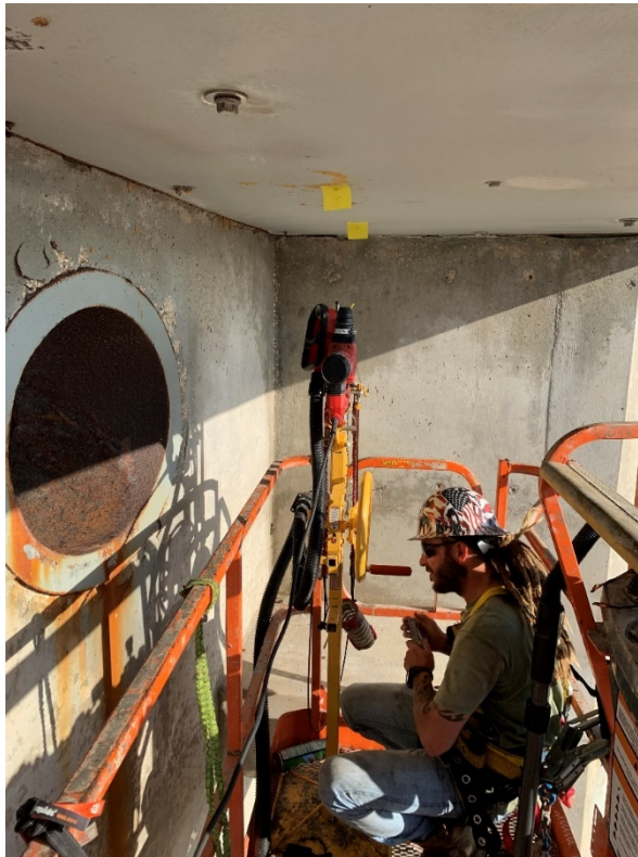
Figure 138: 11/16/2020 3:39:12 PM; preparing to drill anchor hole during "phase 2" of anchor installation
