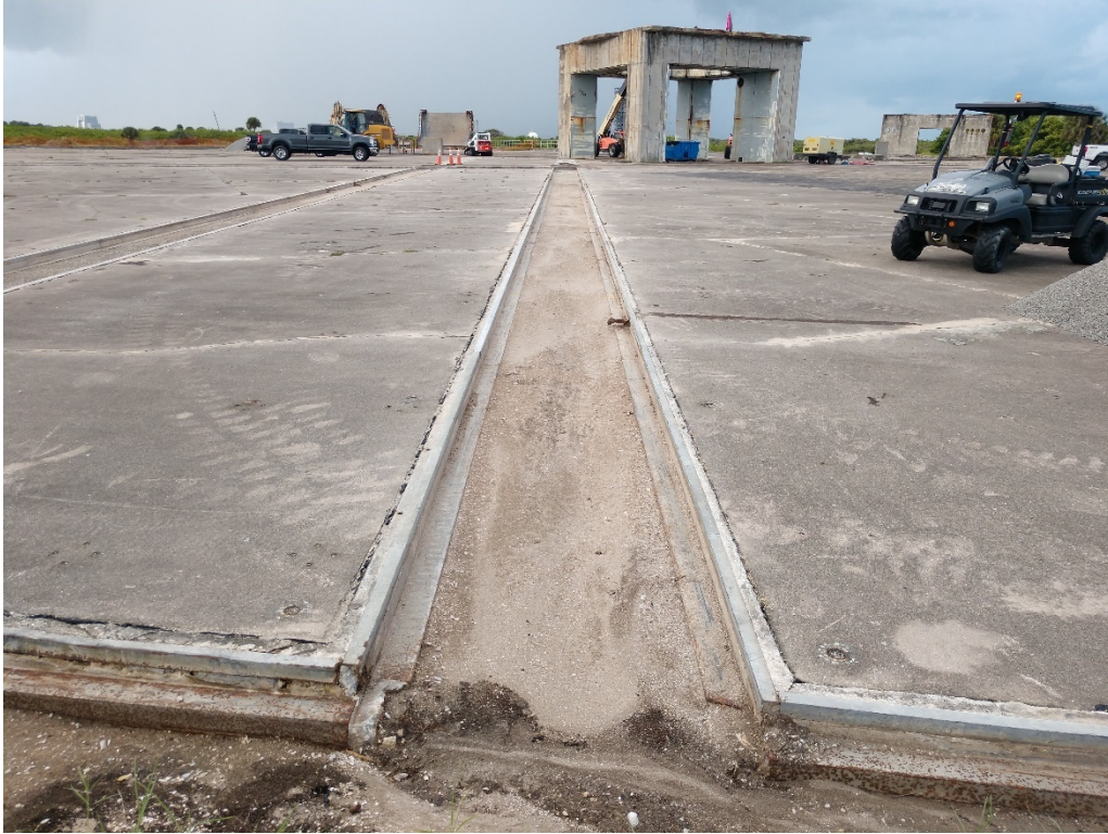
Figure 97: 9/29/2020 3:27:15 PM; facing NW, excavated trench on S side of launch pad
