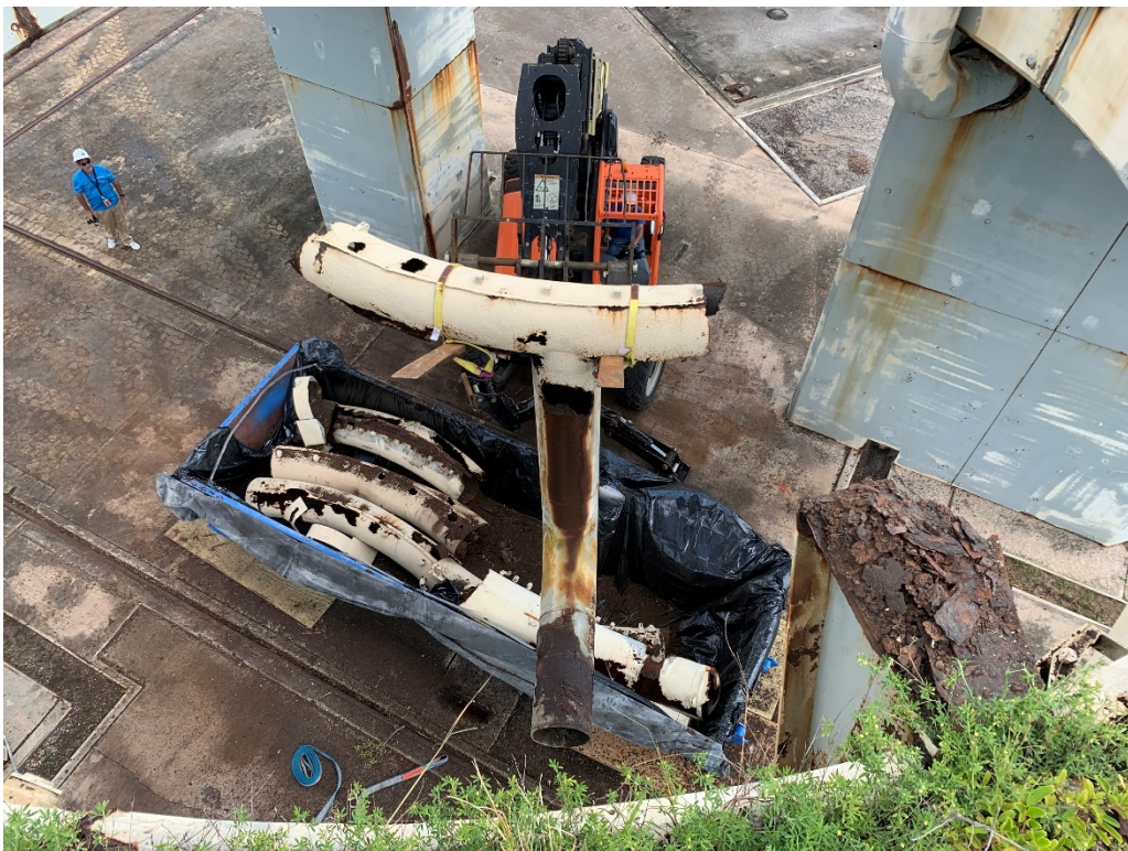
Figure 40: 9/16/2020 10:19:29 AM; lowering Torus Ring section and down pipe
