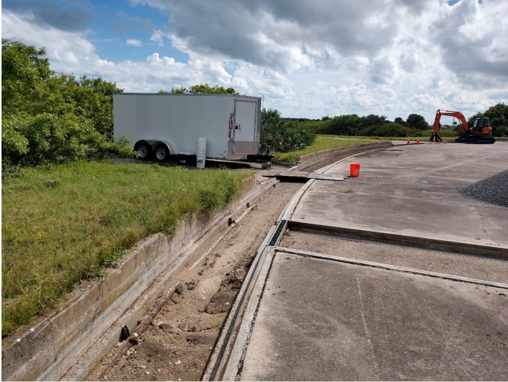
Figure 91: 9/29/2020 3:23:36 PM; facing S, excavated trench on E side of launch pad
