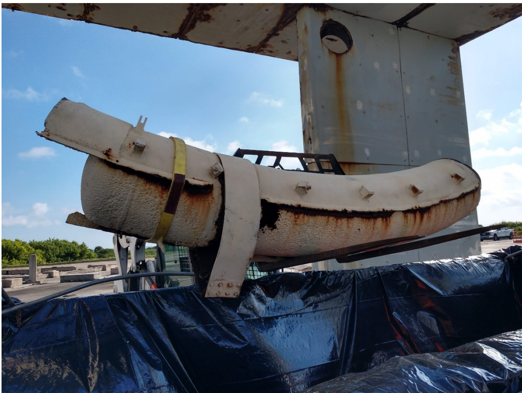
Figure 52: 9/18/2020 10:09:57 AM; Torus Ring section being placed in roll-off box
