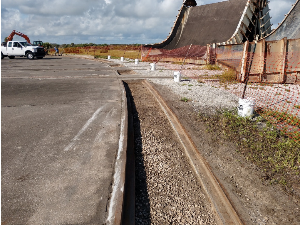
Figure 19: 9/15/2020 9:36:18 AM; facing SW, excavated trenches on NW side of launch pad
