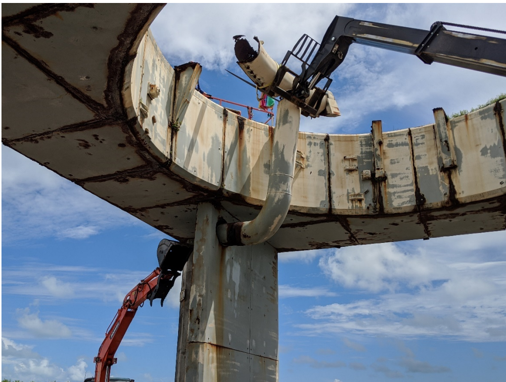
Figure 48: 9/16/2020 1:48:20 PM; removing Torus Ring section and down pipe
