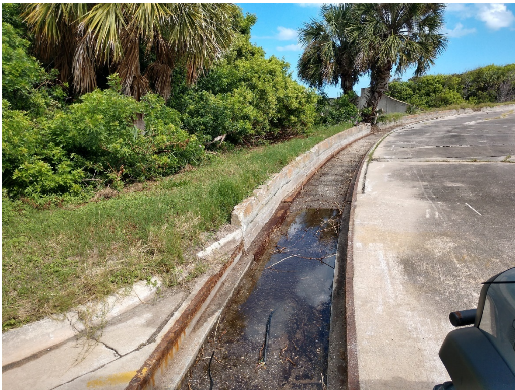
Figure 84: 9/29/2020 3:21:03 PM; facing E, excavated trench on N side of launch pad
