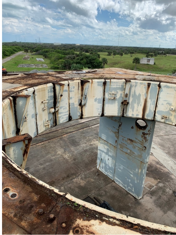
Figure 79: 9/29/2020 3:12:37 PM; top of the Pedestal after sweeping and vacuuming
