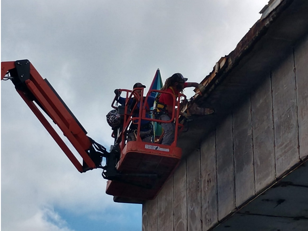
Figure 73: 9/29/2020 11:06:41 AM; removing side edge panels from top of Pedestal
