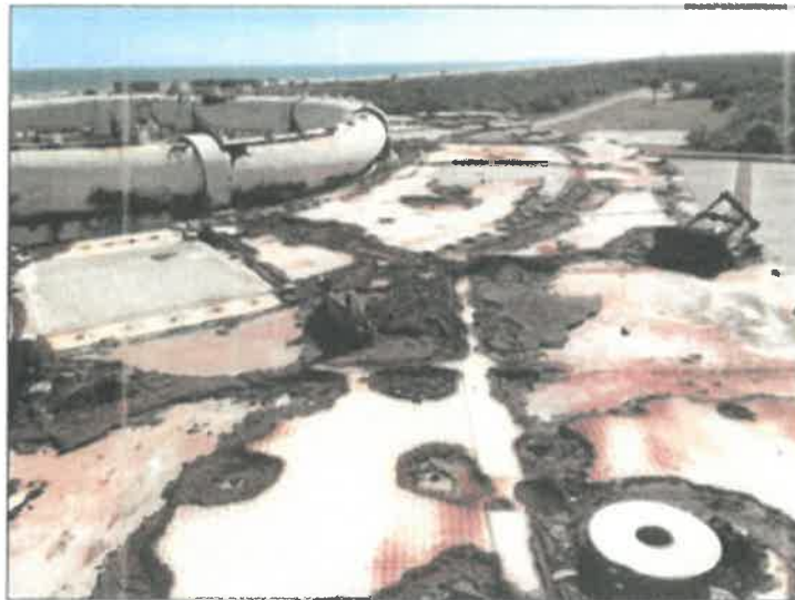
Figure 8. View of the top side of the Launch Pedestal before debris cleanup (2018)
