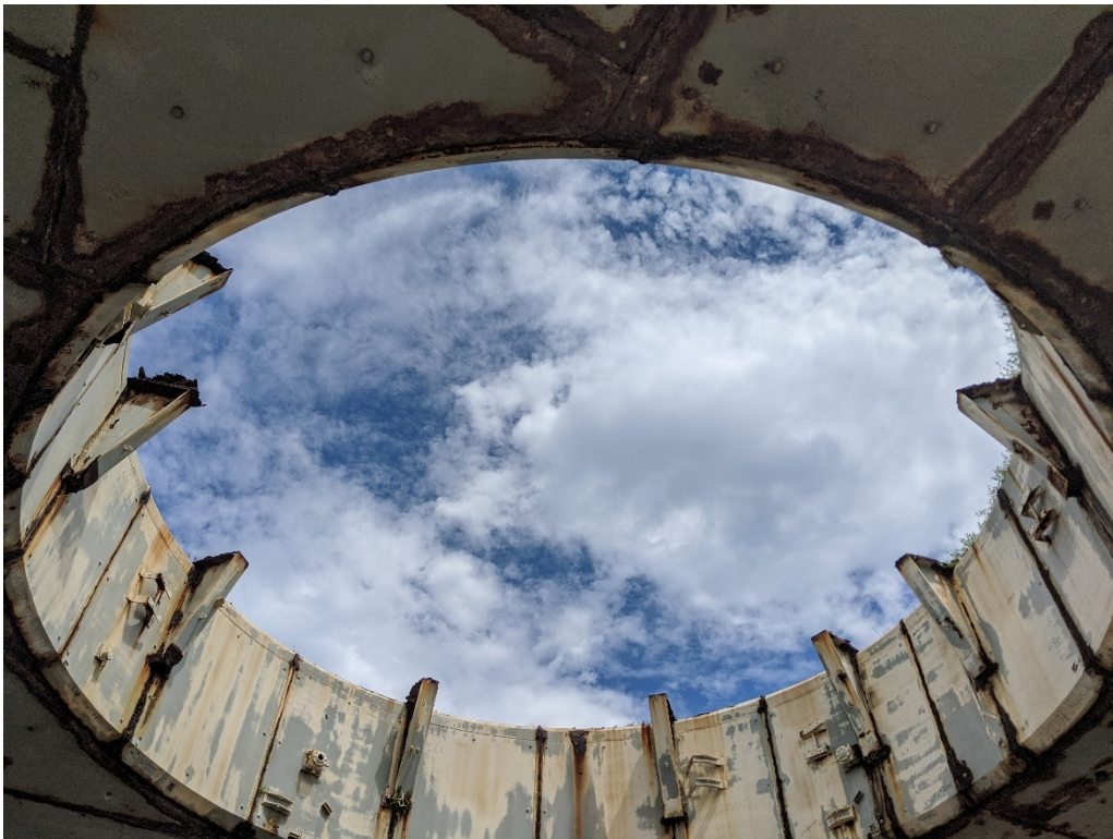
Figure 50: 9/16/2020 1:52:26 PM; looking from underneath Pedestal with Torus Ring removed
