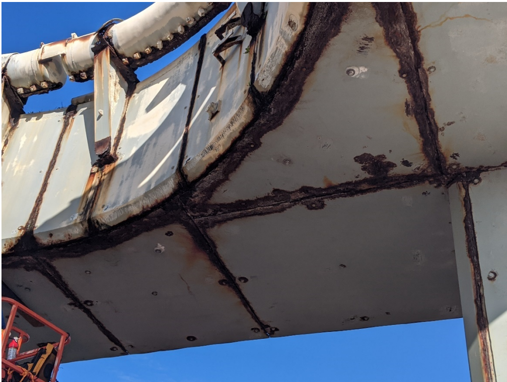
Figure 8: 9/10/2020 8:50:29 AM; looking at underside steel plates with newly installed anchors
