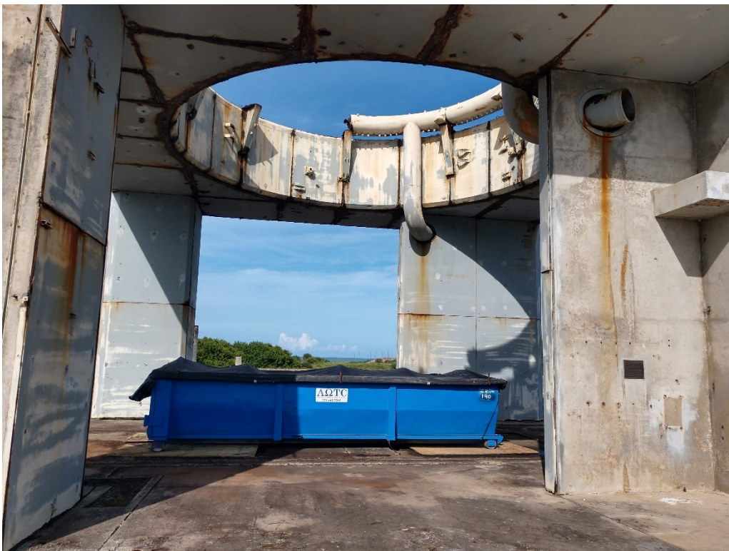
Figure 36: 9/15/2020 4:28:10 PM; looking from underneath Pedestal with sections of Torus Ring removed
