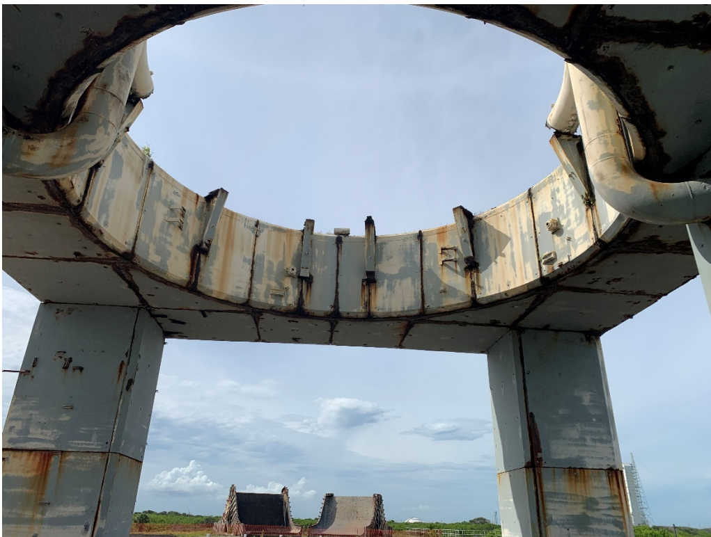
Figure 32: 9/15/2020 3:57:30 PM; looking from underneath Pedestal with sections of Torus Ring removed
