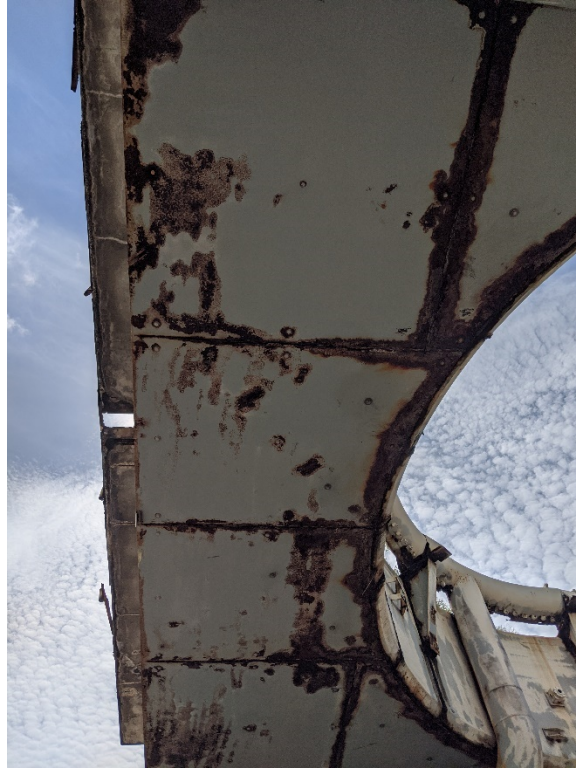
Figure 17: 9/14/2020 2:26:17 PM; looking at underside steel plates with newly installed anchors
