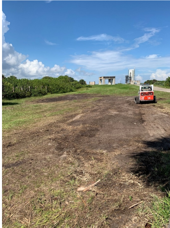
Figure 135: 10/9/2020 1:19:49 PM; restoring excavated soil stockpile to original conditions
