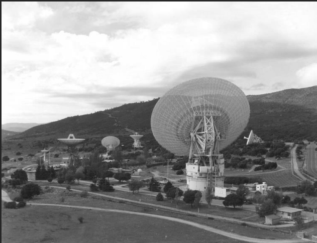
The Robledo de Chavela Station– Received images from Mars transmitted by Mariner 4 – July 1965
