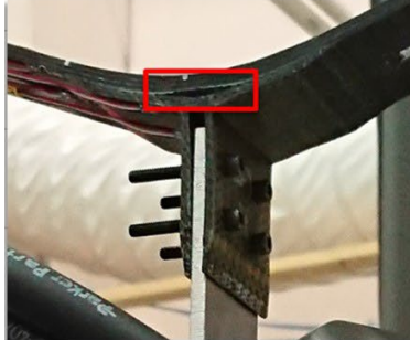
Fig. 1 Initial failure region in the Y-joint as seen in experiments [4].
