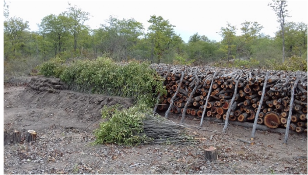
Figure 3: Kiln under construction. Mopane logs in the process of being covered by branches and dirt.
