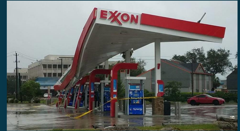
Post-storm damage in Clear Lake, TX Source: NASA/K. Yang
