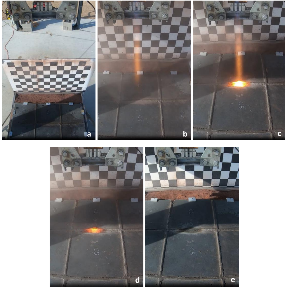
Figure 10. Set of sintered pavers installed over regolith (a) just prior to testing of grout exposure to engine plume, (b) as the engine descends approximately halfway to the stops, (c) glowing while the engine is at its closest position on the stops (60 cm above test article), (d) at engine shutdown, and (e) less than a second after engine shutdown. The offset position of the paver assembly is revealed by the presence of uncovered regolith.
