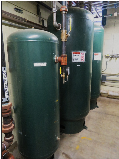
Figure 4.—Left to right: The service air receiving tank and two 93 percent oxygen storage tanks.
