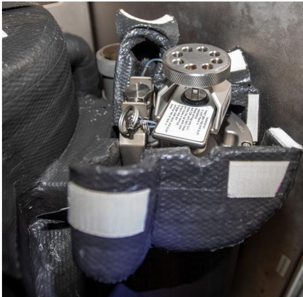
Figure 8. GTPA installed on Node 3 MTL GT
