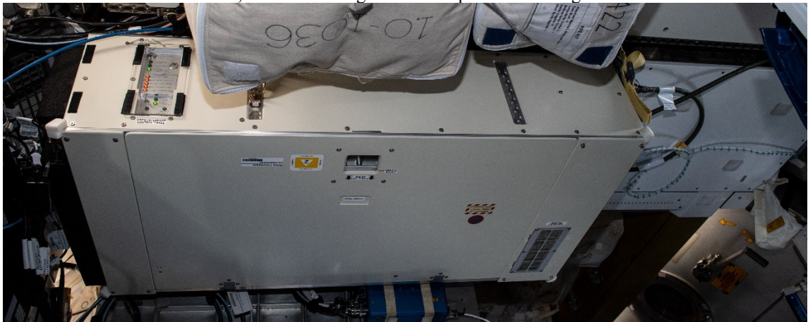
Figure 6. Brine Processor Assembly Installed on ISS.
