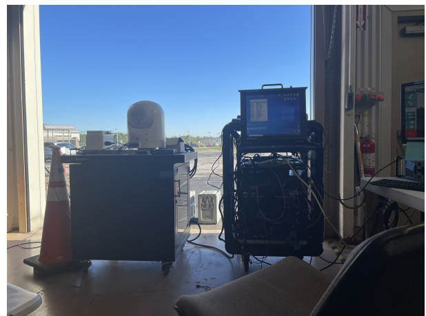
Figure 7. Ground setup of optical modem and transceiver
