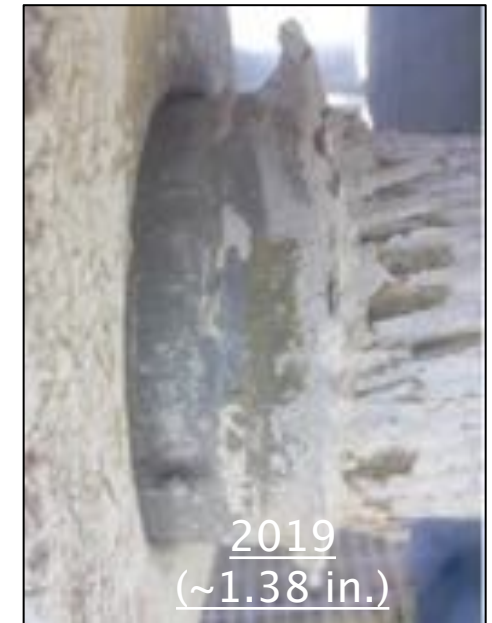
Inspection Photos showing Zinc Extrusion (representative Aux sockets)
