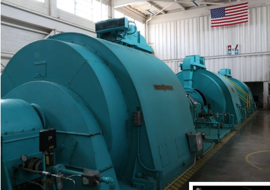
Three 29,000-hp drive motors set in series drive a single shaft
