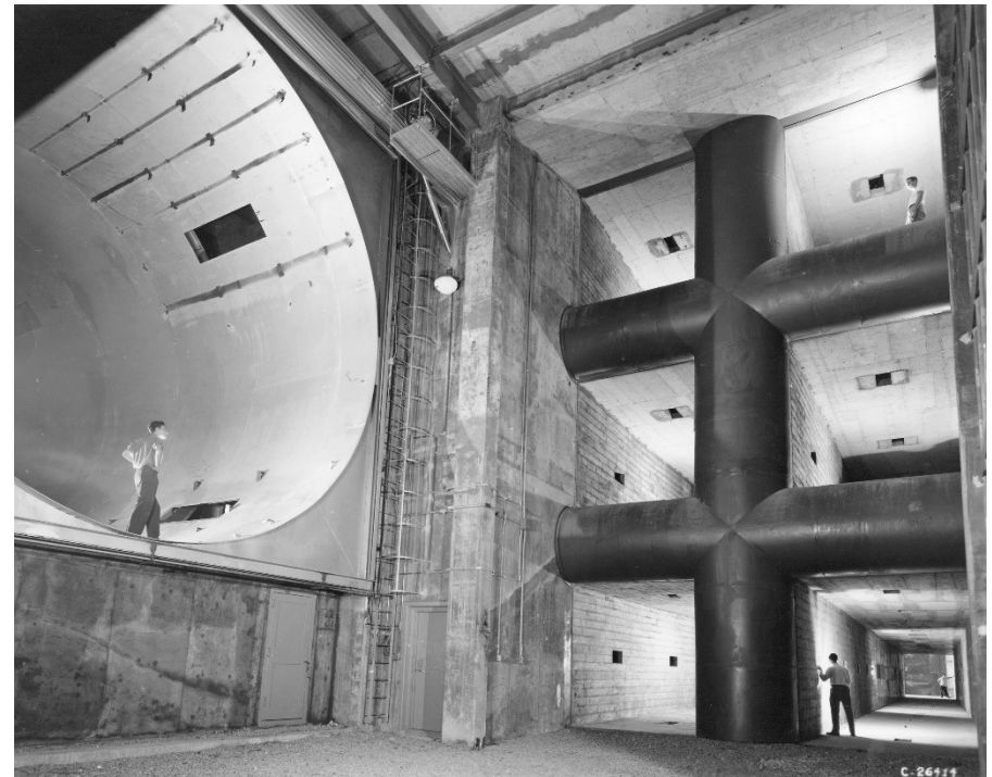
C-1950-26414 End of 8x6 SWT diffuser, into Turn #1, and into triple-storied Acoustic Muffler
