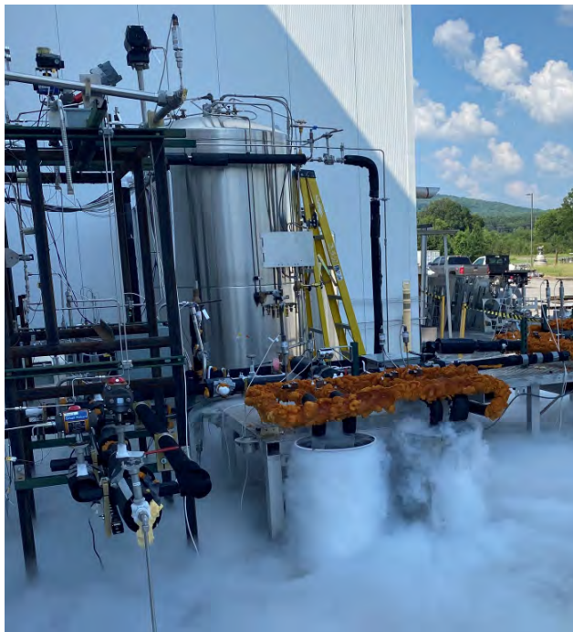
FIGURE 2. IRCS Testbed simulating firing using liquid nitrogen during testing.
