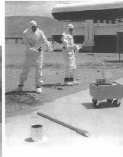
200 hp vacuum cleaner used for small fuel pieces. Reach extender used to get large fuel pieces
