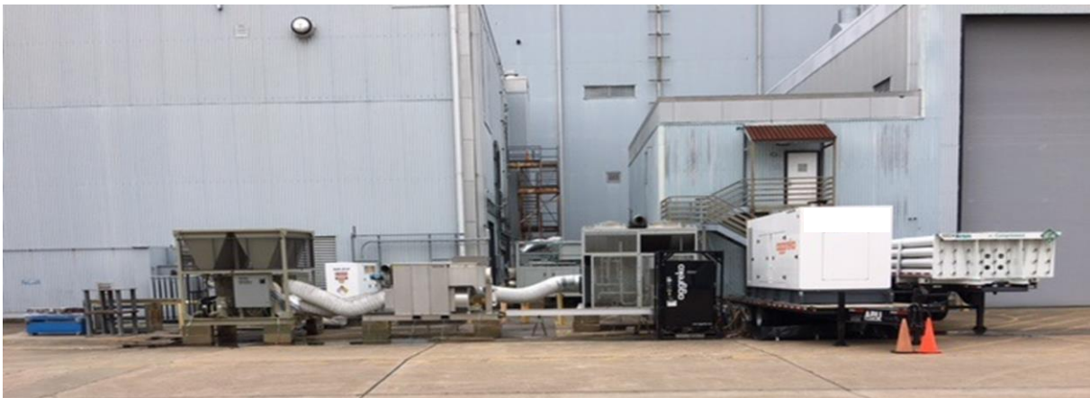
Figure 7. Cleanroom backup AFMS (Photo credit: NASA/Edwin Goldman)
