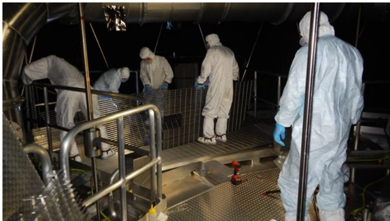
Figure 13. CC technicians cleaning areas under floor grating on level 5 (Photo credit: NASA/Joe Ward)
