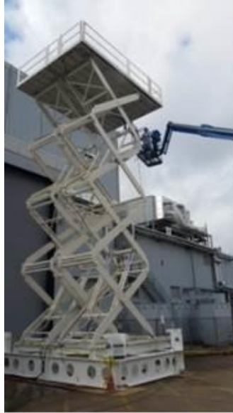
Figure 20. Pentalift inspection just outside the JSC building 32 truck lock (Photo credit: NASA/John Byard)
