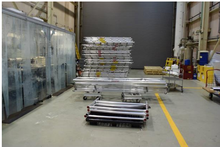
Figure 19. Scaffolding staged in truck lock before ingress into cleanroom and cleaning station on left. (Photo credit: NASA/Joe Ward)
