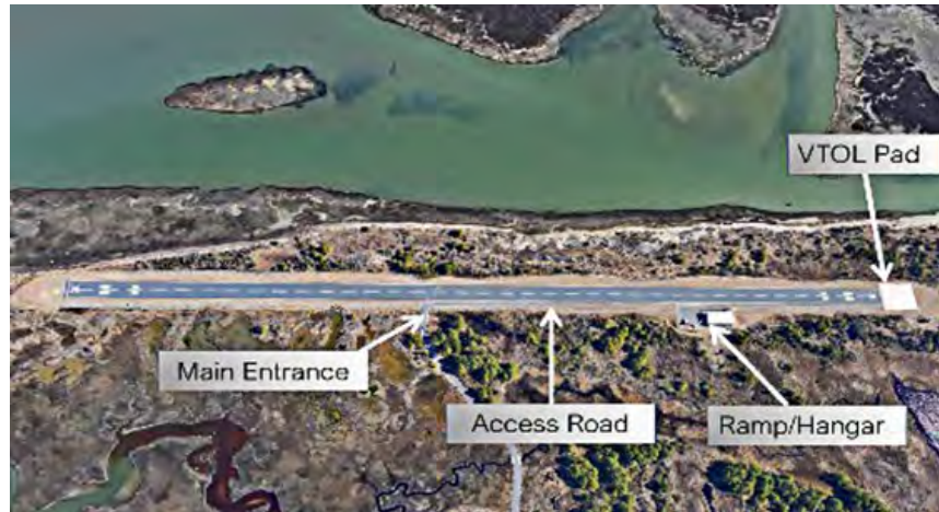
Figure 72: MARS UAS Airfield
