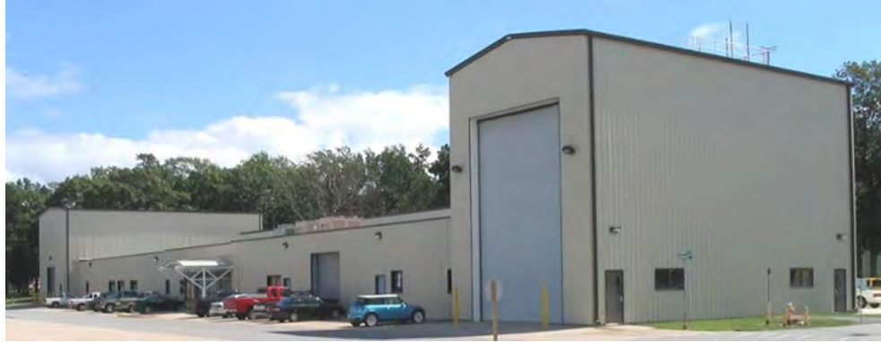
Figure 47: Integration and Test (Building F-7)
