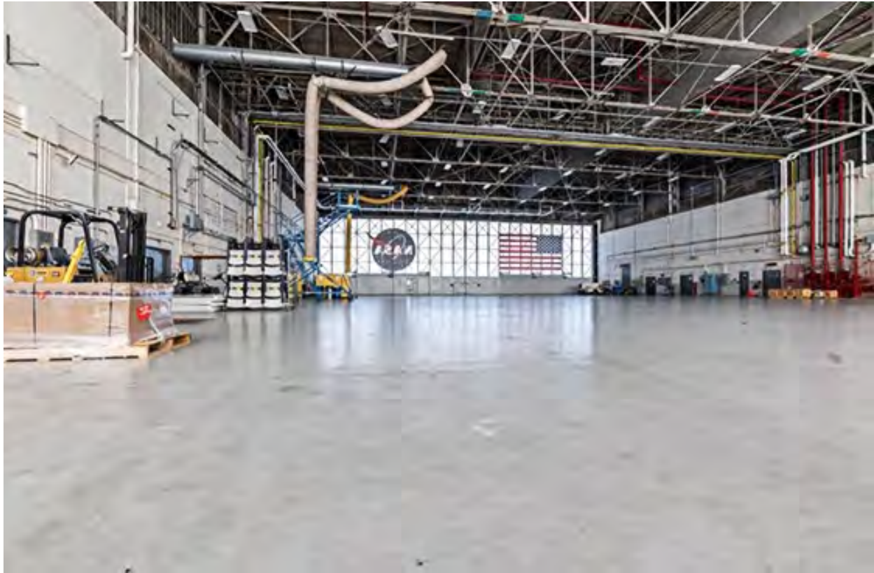
Figure 70: Aircraft Operations Hangar (Building D-1)
