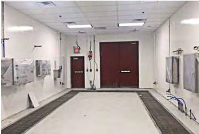
Figure 81: MARS Payload Processing Facility Secondary Payload Processing Bay
