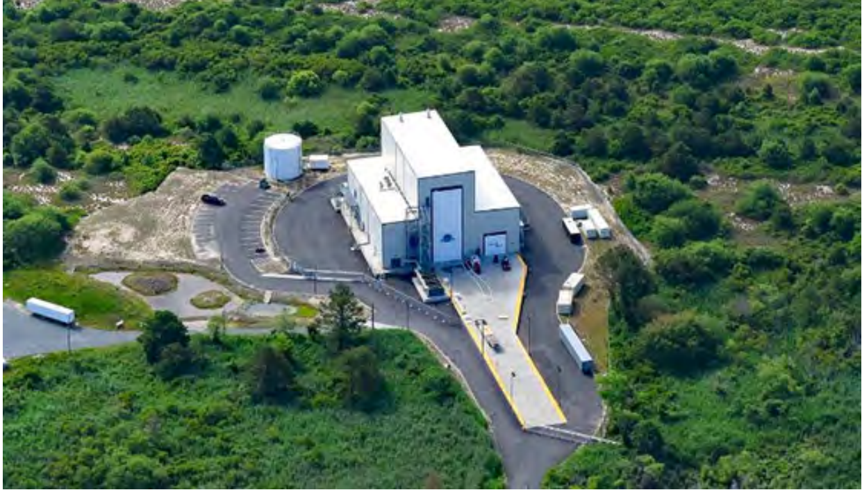
Figure 79: MARS Payload Processing Facility
