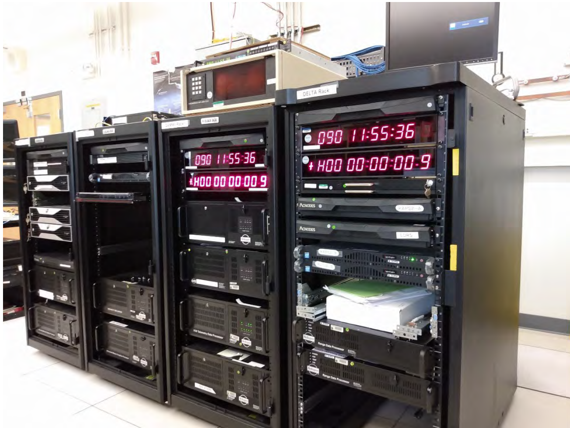
Figure 67: Software Development Lab (Building E-109)
