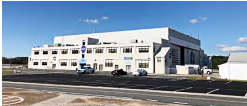
Figure 68: Aircraft Operations Hangar (Building D-1)
