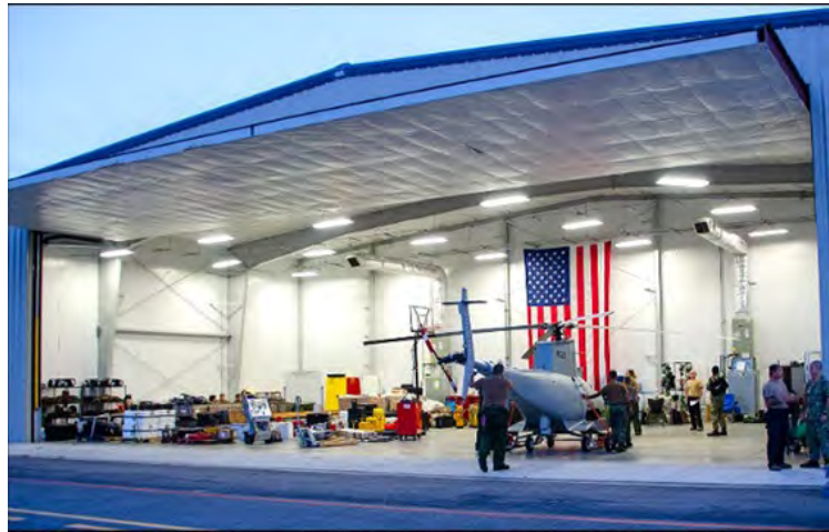
Figure 75: MARS UAS Airfield HVAC Conditioned Hangar
