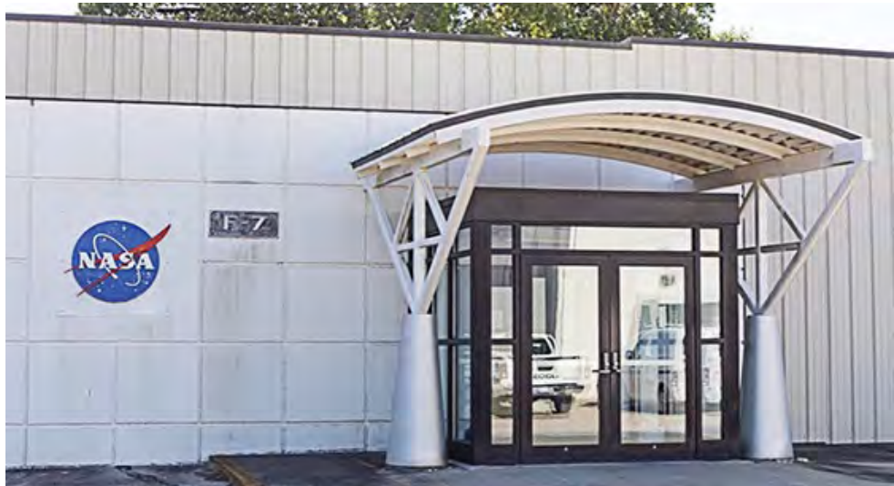
Figure 48: Integration and Test (Building F-7)
