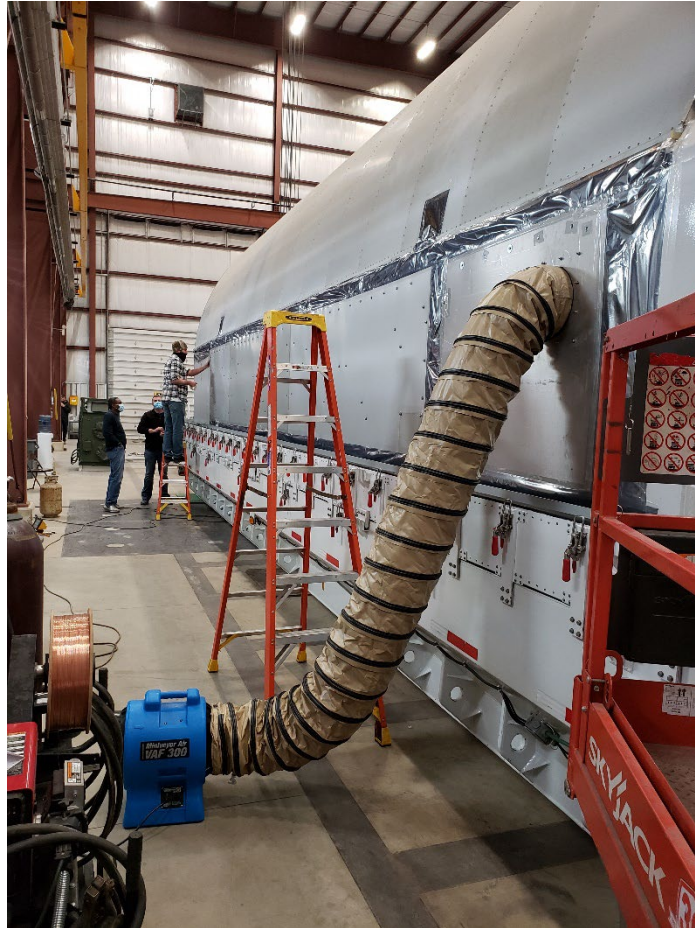
Figure 9. Leak testing the closeouts at Nelson Manufacturing. (Credit: Joseph Ward)
