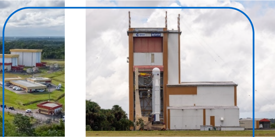
S5B BAF Hazardous Processing Facility
