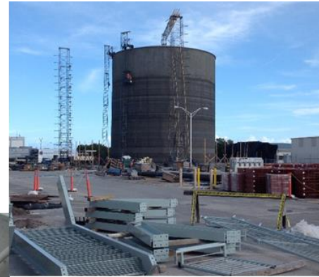
Tank Being Wrapped
