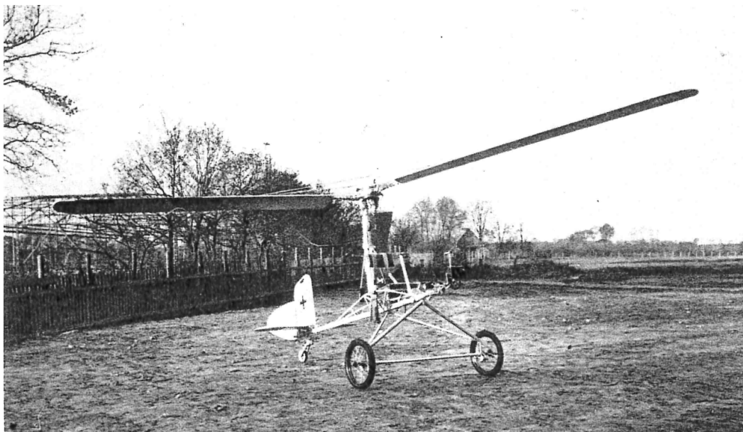
Fig. 28: Fa 330. Small gyroplane that can be taken apart for submarines.
