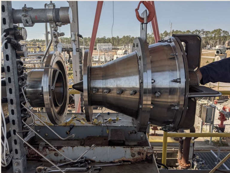
Side view during installation.
