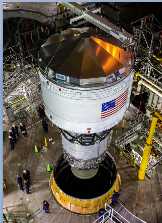
Above: ICPS mating with SLS core stage. Right: Multiple interfaces exist between the ML and the Artemis I vehicle. The crew access arm and Orion service module umbilical are located at 280 feet, the ICPS umbilical complex is next at 240 feet, followed by the vehicle stabilizer system and the core stage forward skirt umbilical at 200 and 180 feet, respectively.
