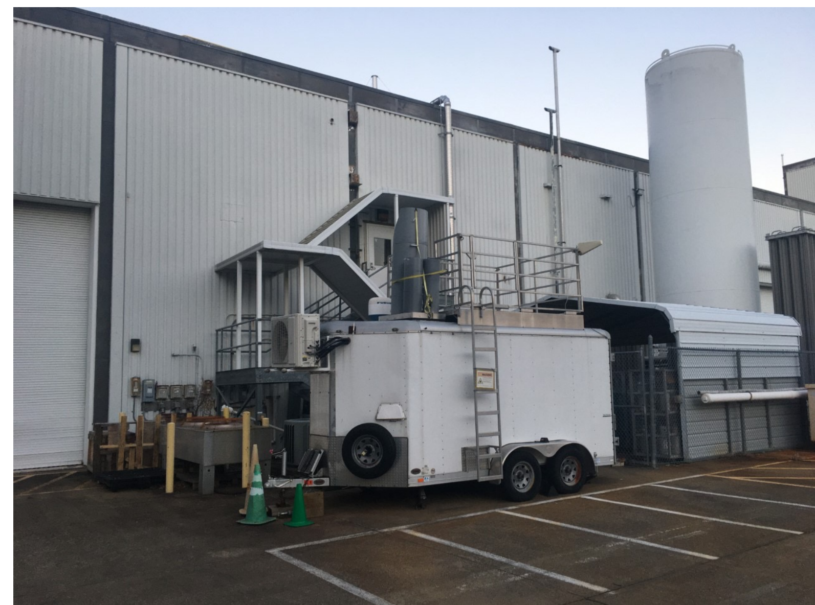
LMOL parked behind the Atmospheric Science building (B1250) at NASA Langley Research Center
