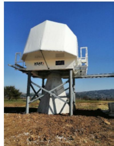
Figure 11.37: KSAT's low-complexity optical ground station in Nemea (2021).
