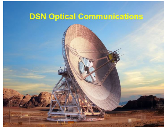
Figure 11.36: Artist overlay of built DSN RF antenna and planned 8m optical segments at its center. Credit: NASA.
