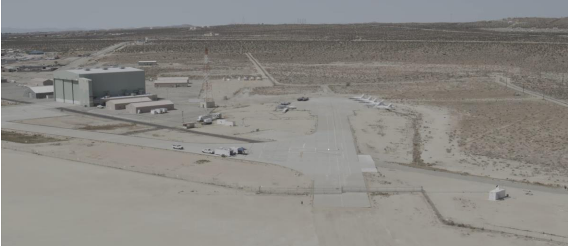
Figure 13. Flight image captured over the AFRC vertiport facility.
