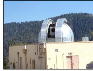
OCTL Ground Station
