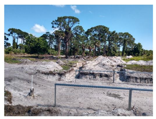
Figure 9: 4/7/2020 3:49:28 PM; Looking southwest, erected pipe racks in manifold trailer area and excavated trenches for Zones 6, 7, and 8 lateral piping.
