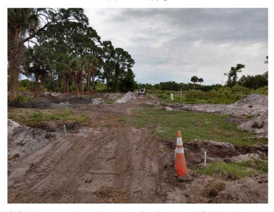
Figure 10: 4/10/2020 3:27:11 PM; Looking south, spreading trench spoils to prepare path for deploying late piping in Zones 6, 7, and 8.
