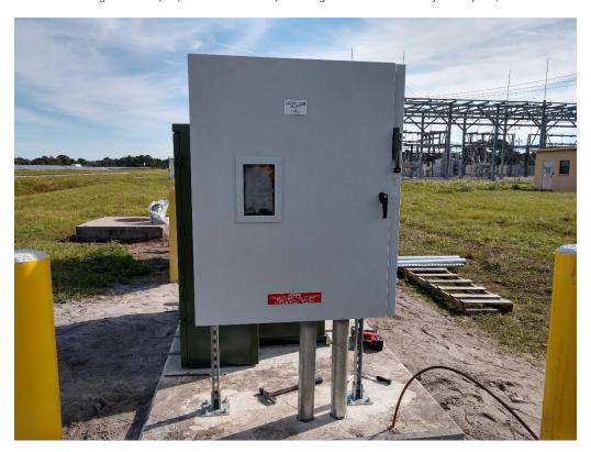
Figure 36: 12/10/2020 11:08:53 AM; Installed and anchored disconnect on transformer pad.
