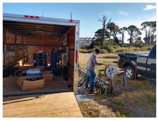
Figure 42:  $1/11/2021\ 10:10:52\ AM$ ; Looking east, installing  $\frac{1}{2}$ -inch flex hose to connect laterals to the legs within the manifold trailer.
