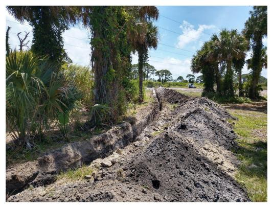
Figure 24: 5/15/2020 2:26:55 PM; Looking southwest, excavated trench for placement of header piping.
