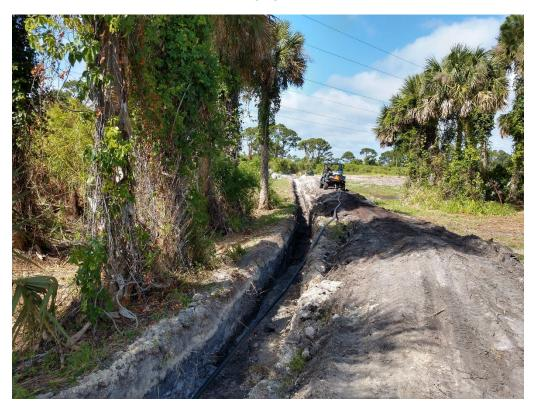
Figure 26: 5/19/2020 10:05:25 AM; Looking southwest, deployment of 2-inch HDPE header piping.
