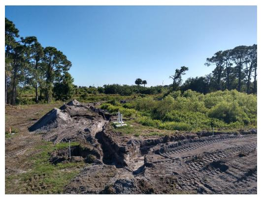
Figure 4: 3/20/2020 4:40:37 PM; Looking south, excavated trenches for Zones 6, 7, and 8 lateral piping.
