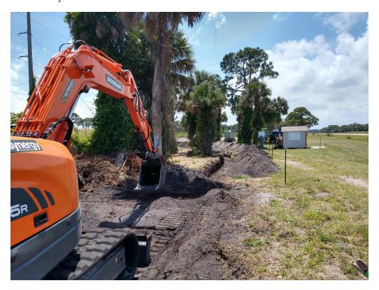
Figure 23: 5/15/2020 2:26:14 PM; Looking west, excavation for placement of header piping.
