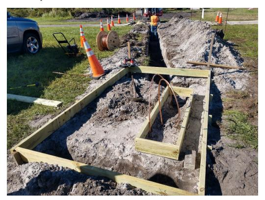
Figure 31:  $11/24/2020\ 10:30:27\ AM$ ; Looking west, excavation of electrical conduit trench and placement of formwork for transformer pad.
