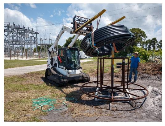
Figure 28: 5/19/2020 2:15:52 PM; Adding a new spool of 2-inch HDPE piping to pipe reel for deployment.
