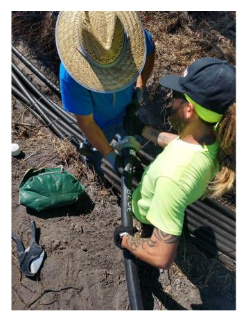
Figure 29: 5/20/2020 10:25:21 AM; Welding 2-inch HDPE header piping with hot plate.
