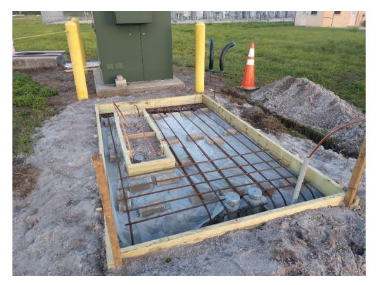
Figure 33: 11/24/2020 4:28:29 PM; Rebar reinforcement in transformer pad.
