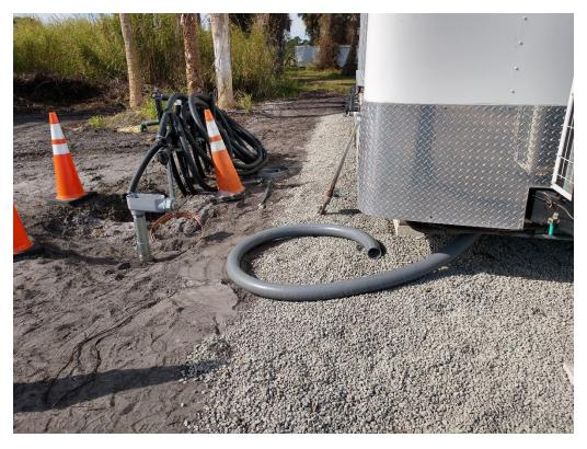
Figure 37: 12/10/2020 11:09:42 AM; Installing flexible conduit to tie rigid conduit to the air sparge trailer.
