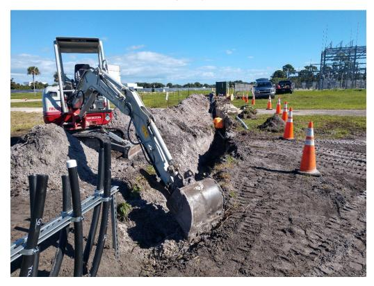
Figure 32: 11/24/2020 11:46:54 AM; Looking east, installation of electrical conduit and ground wire.
