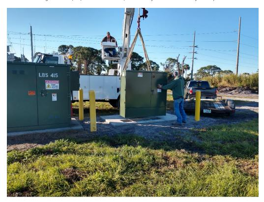
Figure 34: 12/9/2020 8:48:03 AM; Placing transformer on transformer pad.
