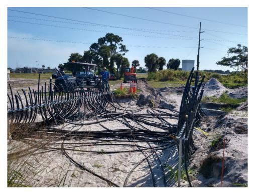
Figure 30: 5/21/2020 9:37:07 AM; Looking northeast, backfilling and placement of warning tape and wire in header trench.
