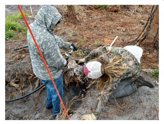
Figure 13: 4/16/2020 12:10:07 PM; Welding 1-inch HDPE lateral to tee for connection to air sparge well.
