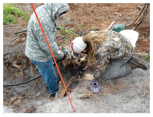
Figure 14: 4/16/2020 12:10:21 PM; PVC gluing 1-inch lateral to tee to air sparge well.
