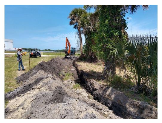
Figure 25: 5/15/2020 2:27:11 PM; Looking east, excavated trench for placement of header piping and installation of barricade signage.
