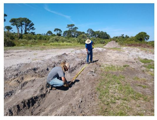
Figure 22: 5/12/2020 10:14:00 AM; Looking west, placement of warning tape and wire in partially backfilled trenches.
