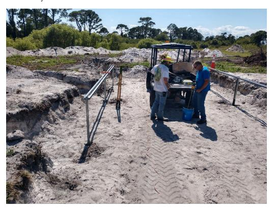
Figure 7: 4/7/2020 3:24:09 PM; Looking west, mixing concrete for setting pipe racks in manifold trailer area.
