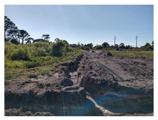
Figure 5: 3/20/2020 4:42:10 PM; Looking west, excavated trenches for Zones 6, and 7 lateral piping.
