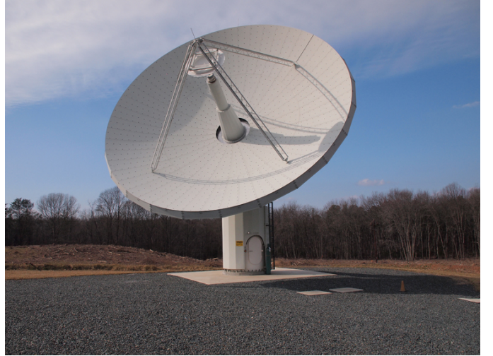
Fig. 1. Photo of the 12 m GGAO VGOS antenna (courtesy of NASA SGP)
