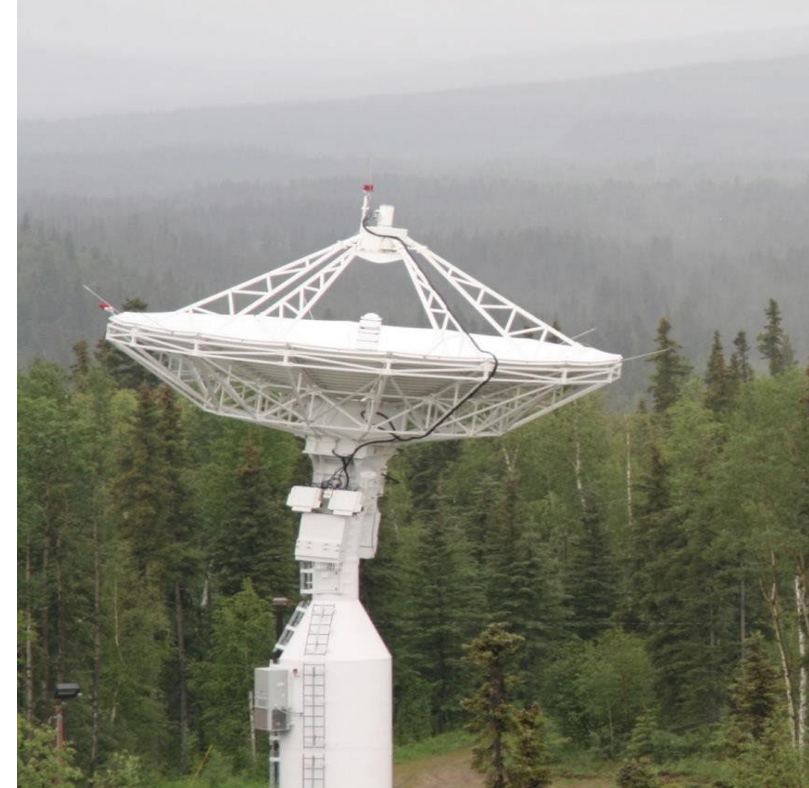
ALASKA SATELLITE FACILITY (NEN)
