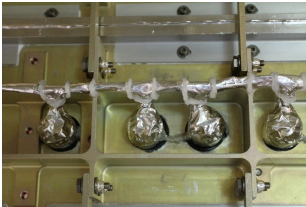
Thermostats Installed on Panel
