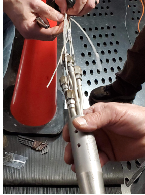
Fig. 12 Hookup of the cap assembly to the pressure lines running from the tunnel measurement system [Source: NASA].
