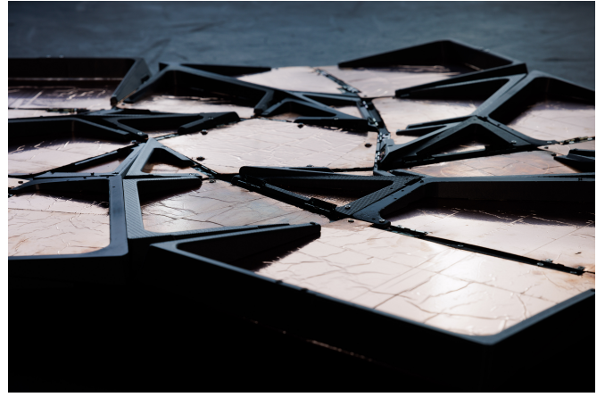
Fig. 5. A close-up view highlights the non-intuitive panel geometry formed as a result of implementing highly structured thickness accommodations. Thin copper wafers align throughout the array to form a coplanar surface.
