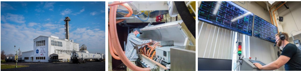
Figure 5. NEAT Facility Exterior, Electrical System Hardware, and Control Room
