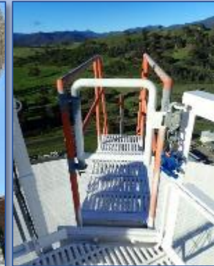
New Access Gate at Apex
