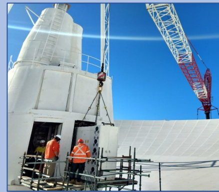
S400 klystron cabinet removal
