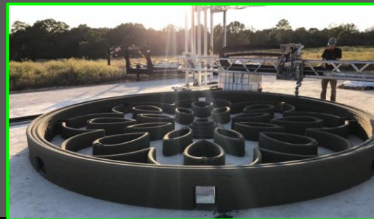
Terrestrial printing of cementitious material
