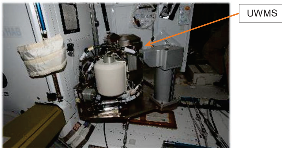
Figure 6.0-1. UWMS Installed in Node 3 on ISS
