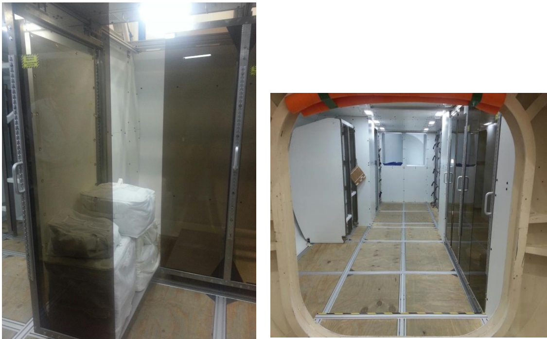
Fig. 46: Final One-G System Installed at MSFC
