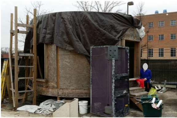
Figure 11. HAVEN habitat exterior before refurbishment
