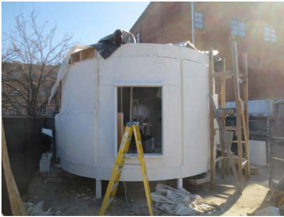
Figure 4. Exterior of HAVEN habitat under construction
