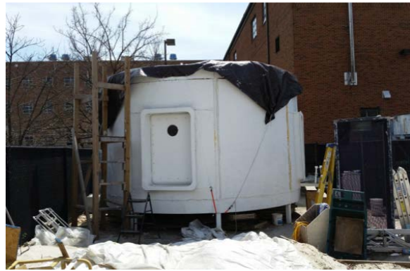
Figure 12. HAVEN habitat exterior after refurbishment
